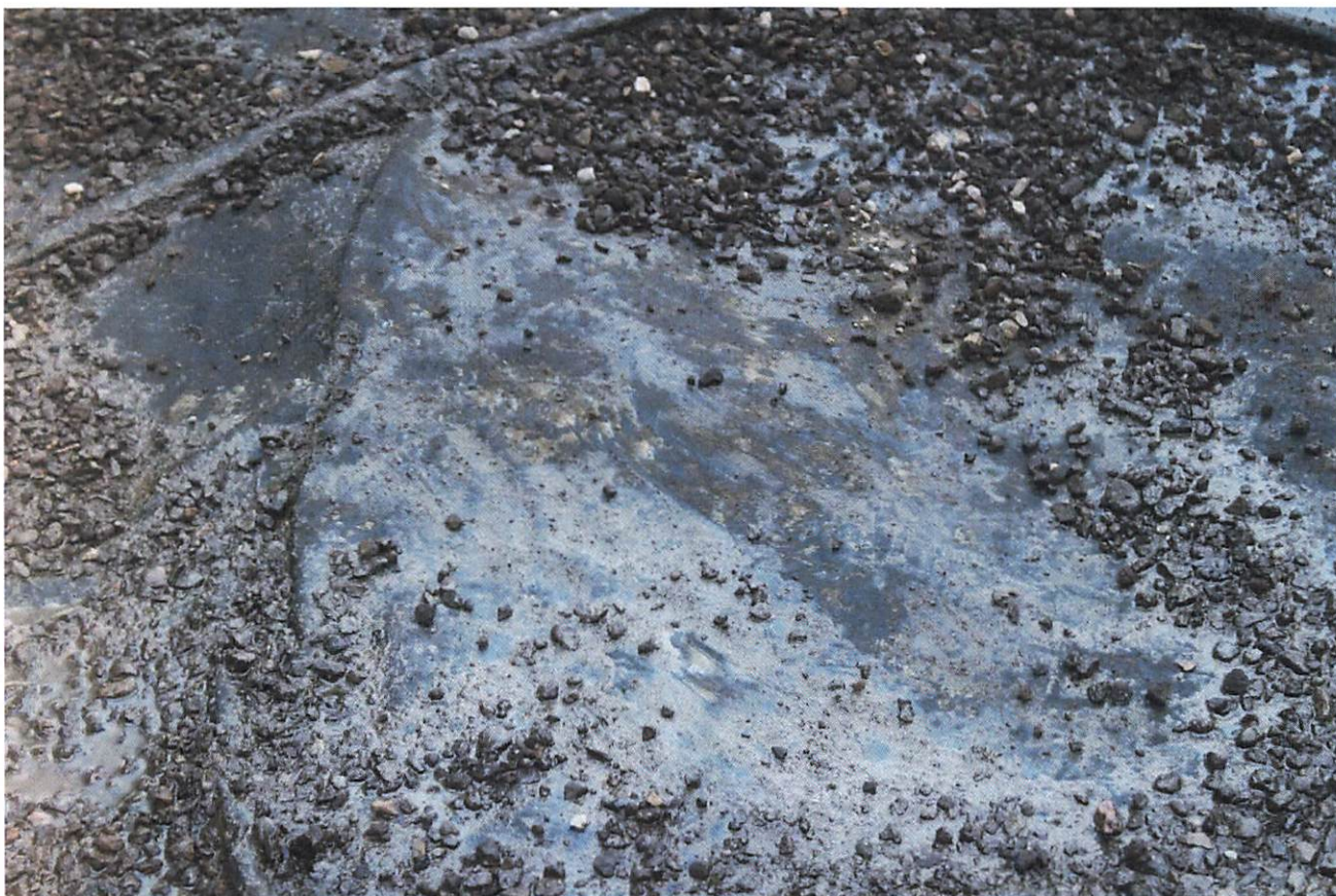
Close-up of liner. Liner is in good shape.
