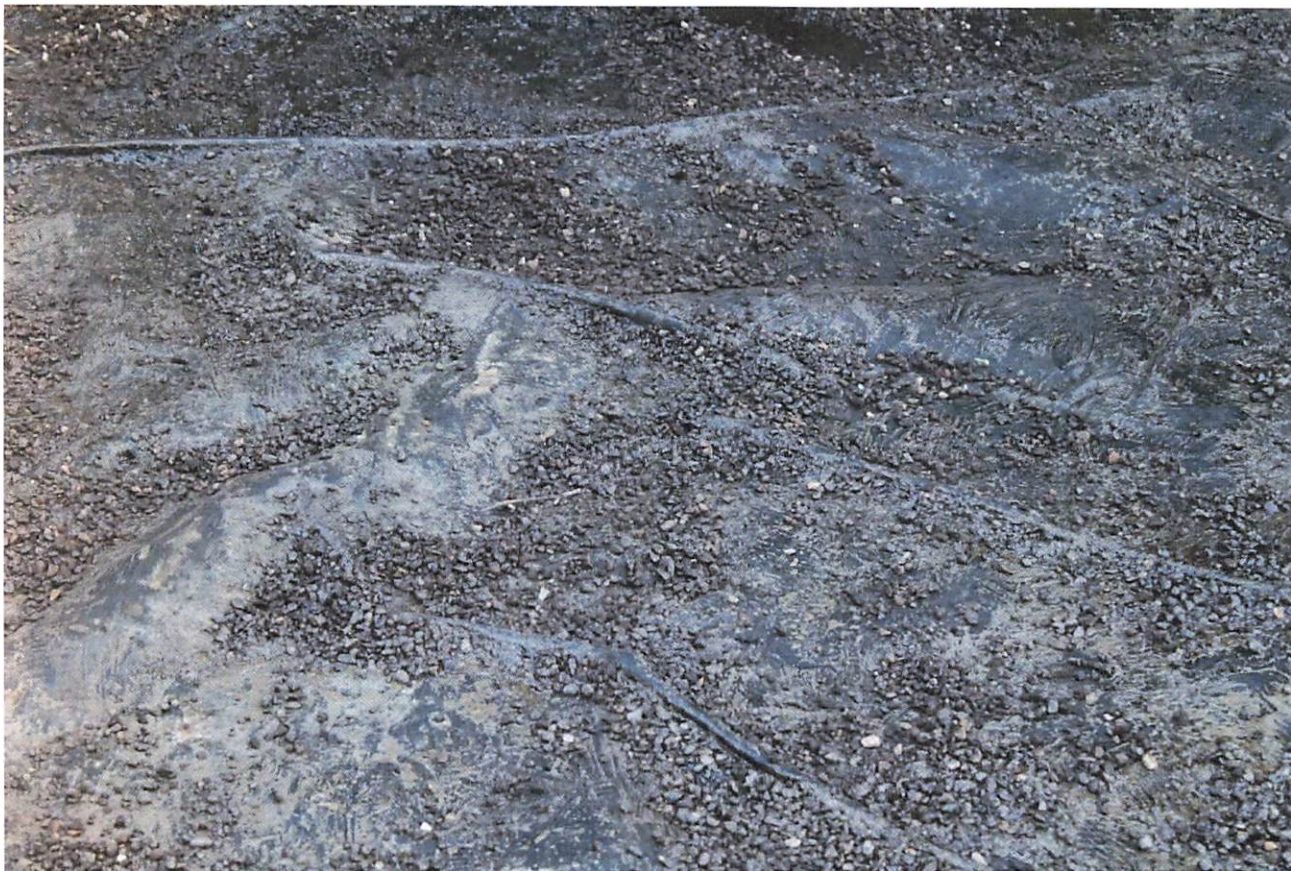
Another location/view of liner. No holes or tears.
