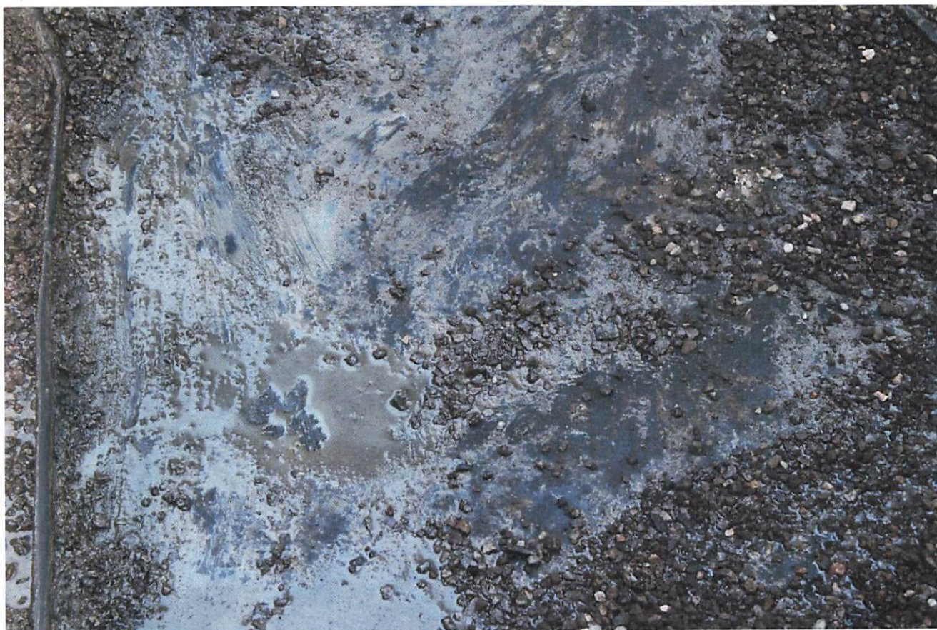
Another location/view of liner. No hole or tears. Liner is holding water.
