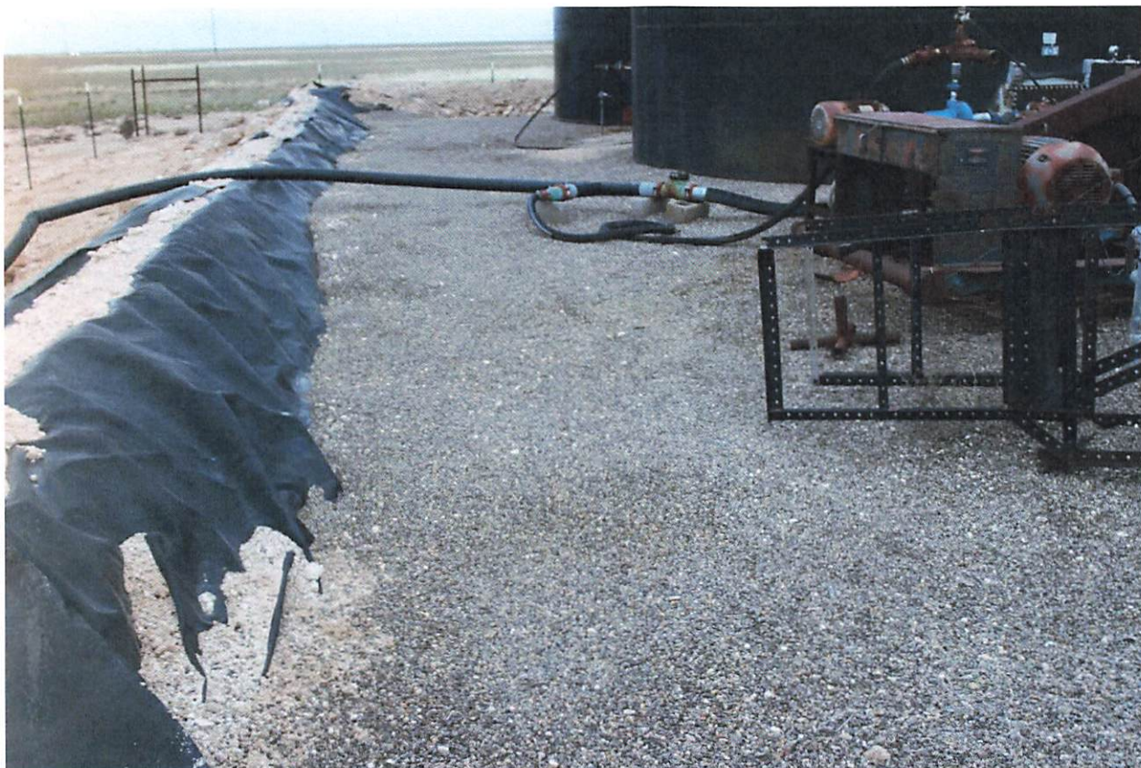
East side of berm facing South. Visible exposed Liner is in good shape.
