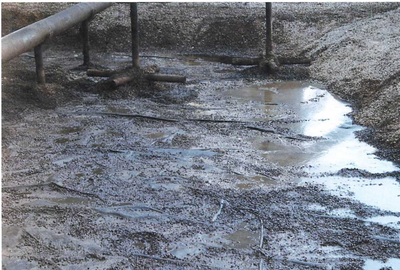
Area where gravel was removed for inspection. Liner is holding water from recent tank washing and some rainwater.
