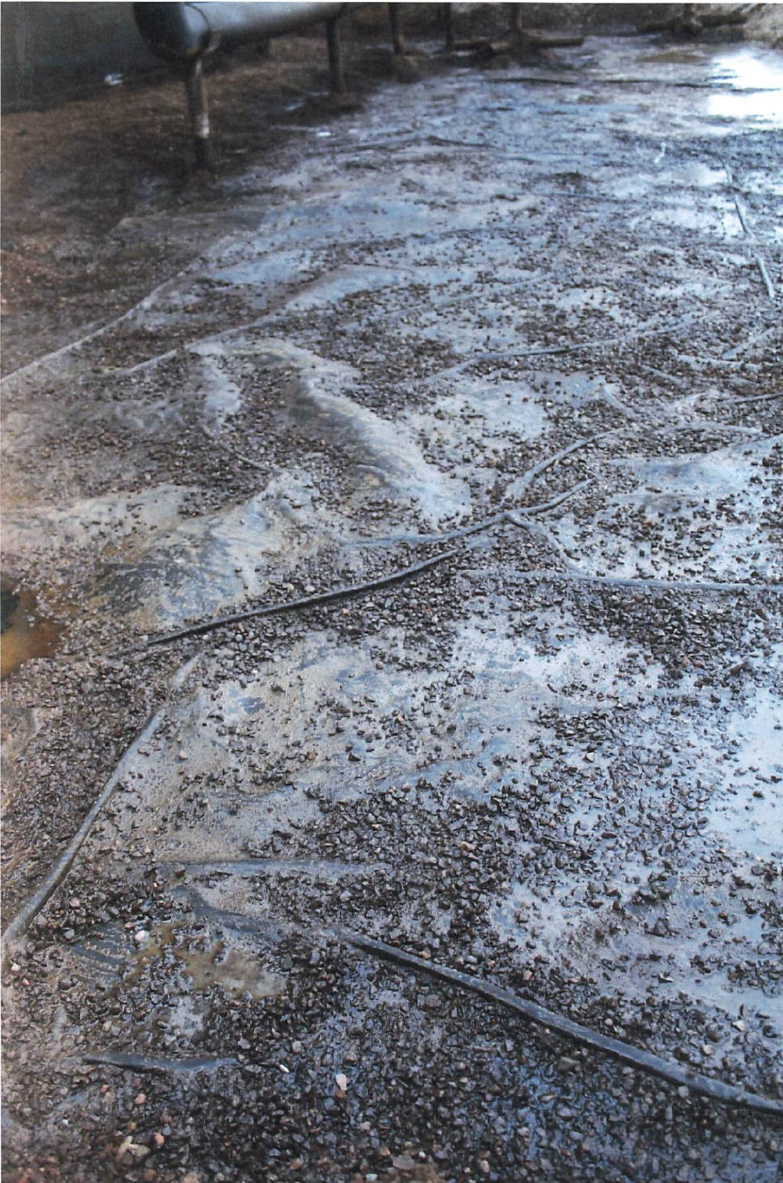
Another view of the exposed liner. Liner is in good shape and holding water.
