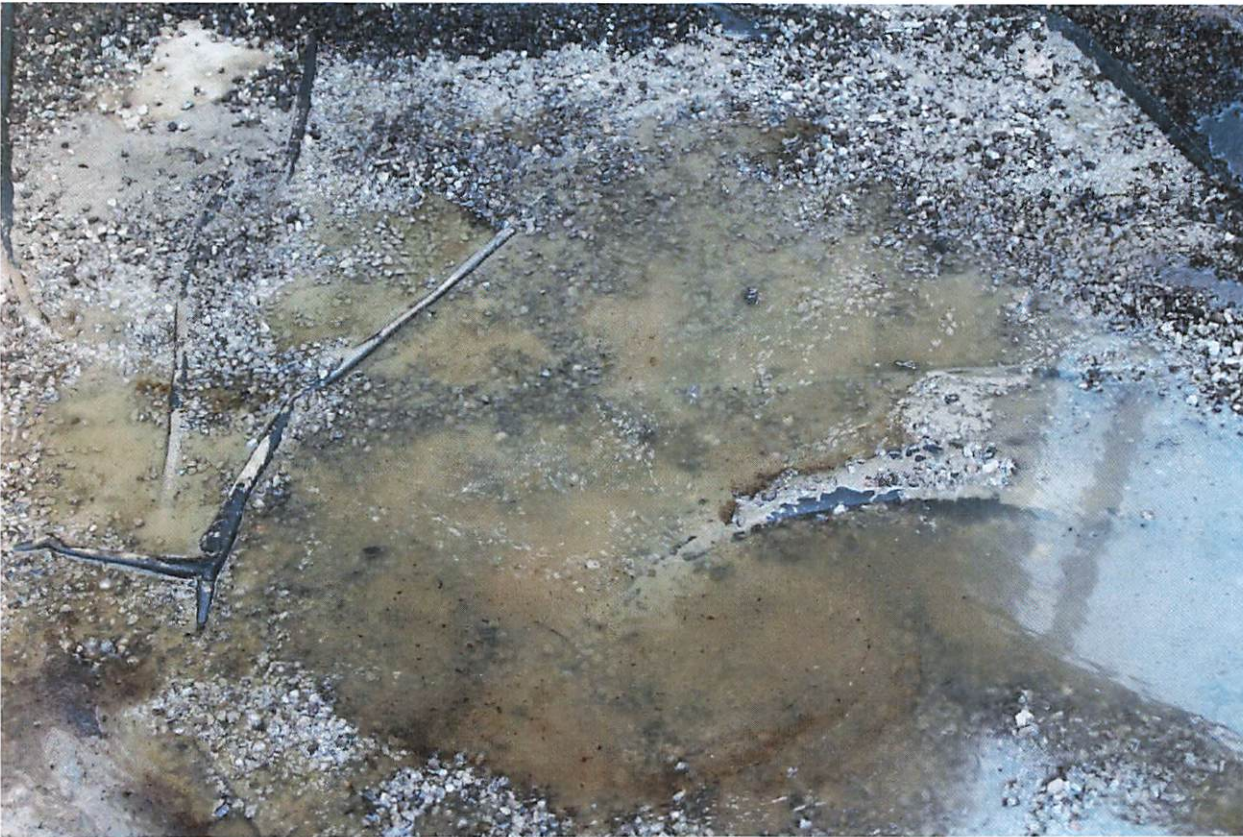
Close-up of liner showing it is holding water.
