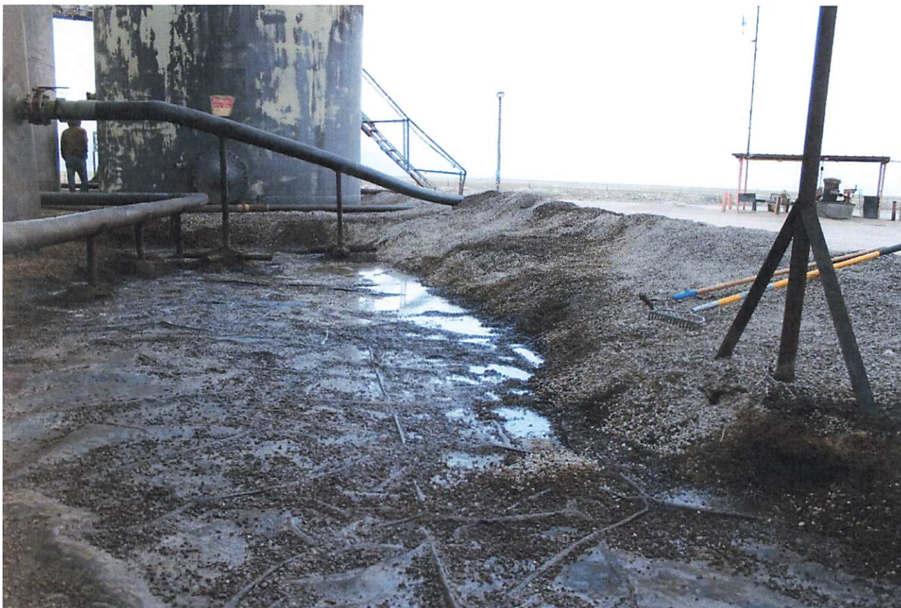
Another view of the exposed liner. Liner is in good shape and holding liquids. Clean gravel will be put back in berm.
