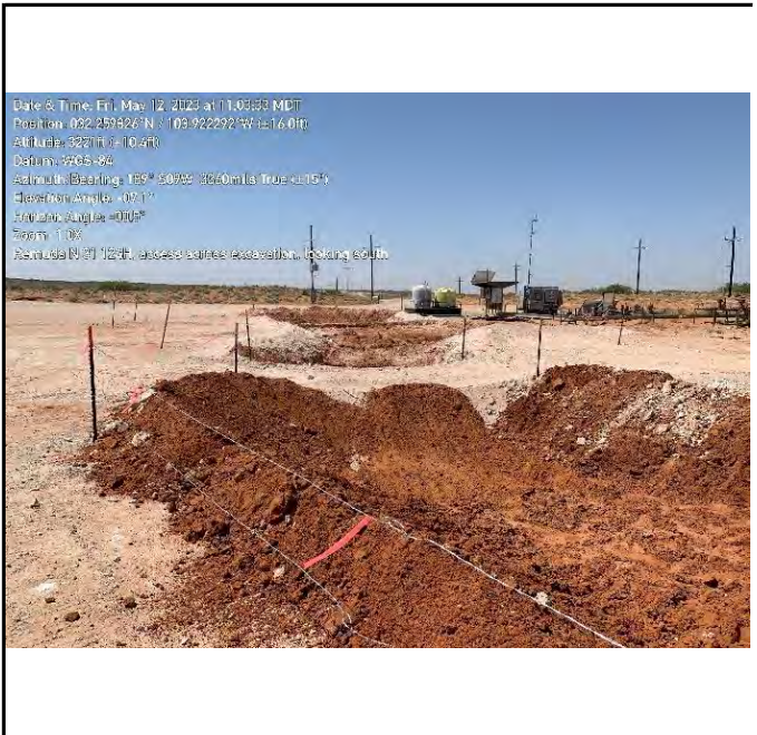
Photograph 4 Date: 05/12/2023 Description: Completed excavation extent on pad View: South
