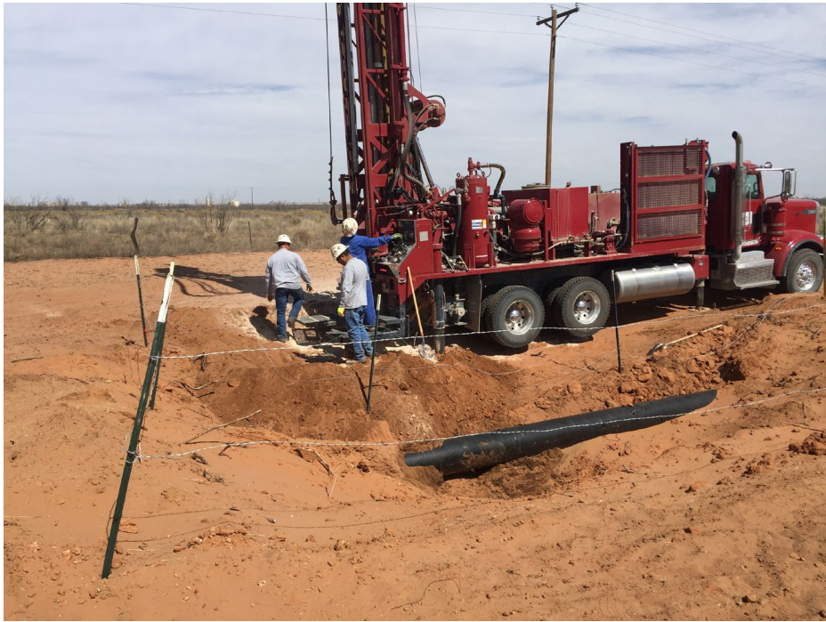
Advancing soil boring SB-2 – 3/8/2018
