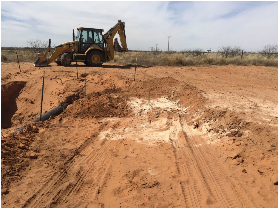
Soil boring SB-2 – 3/8/2018
