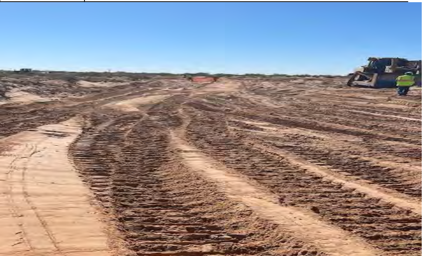
Photo: 2 Description: Backfill
