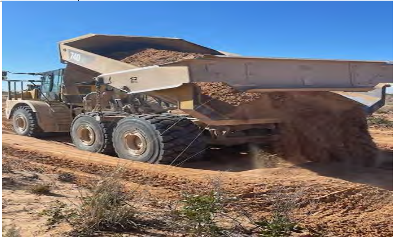
Photo: 1 Description: Backfill
