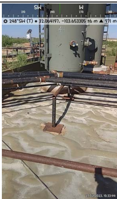
Photograph: 3 Date: 7/27/2023 Description: View of intact liner during inspection
