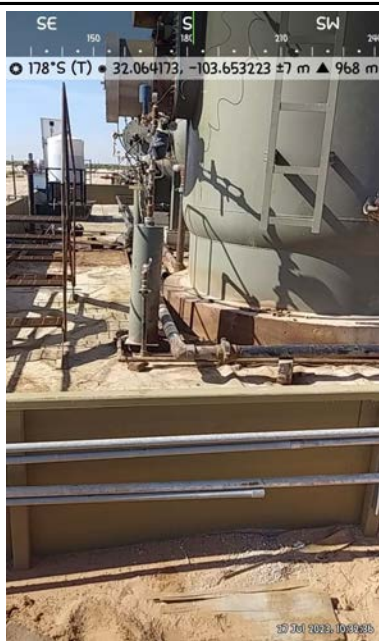
Photograph: 1 Date: 7/27/2023 Description: View of intact liner during inspection
