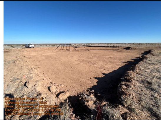
Overview of excavation
