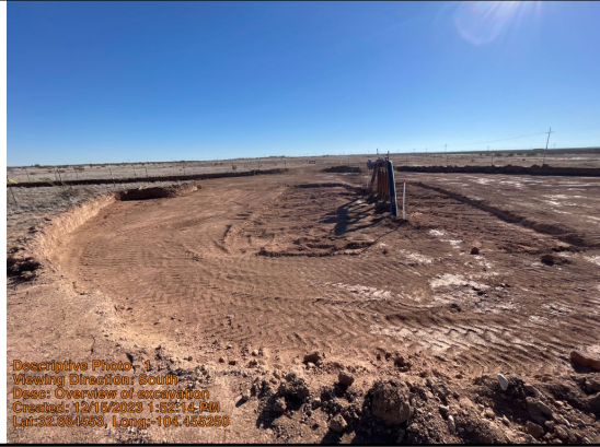
Overview of excavation
