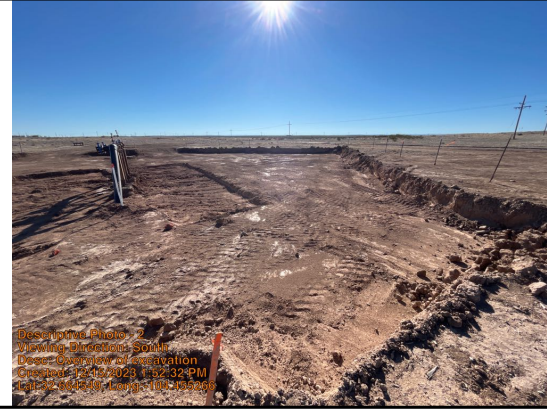
Overview of excavation
