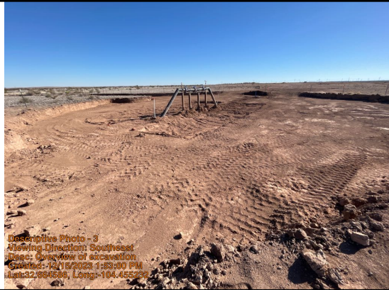
Overview of excavation
