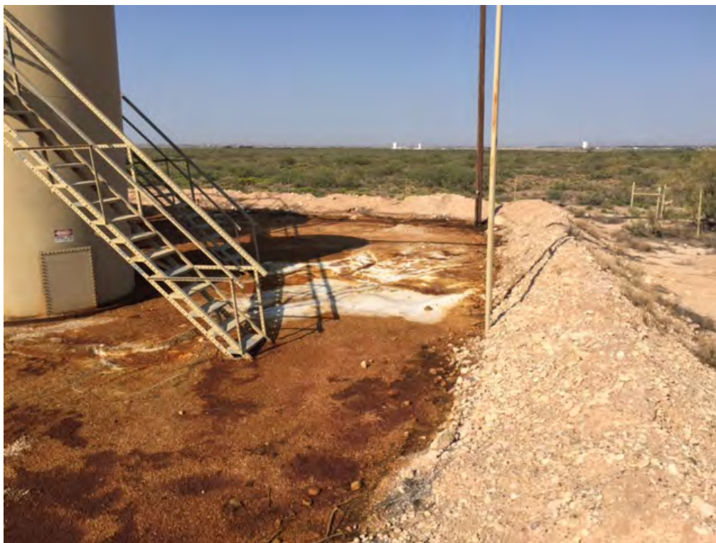
NEL 4 SWD Battery – Release (Looking West-Southwest)
