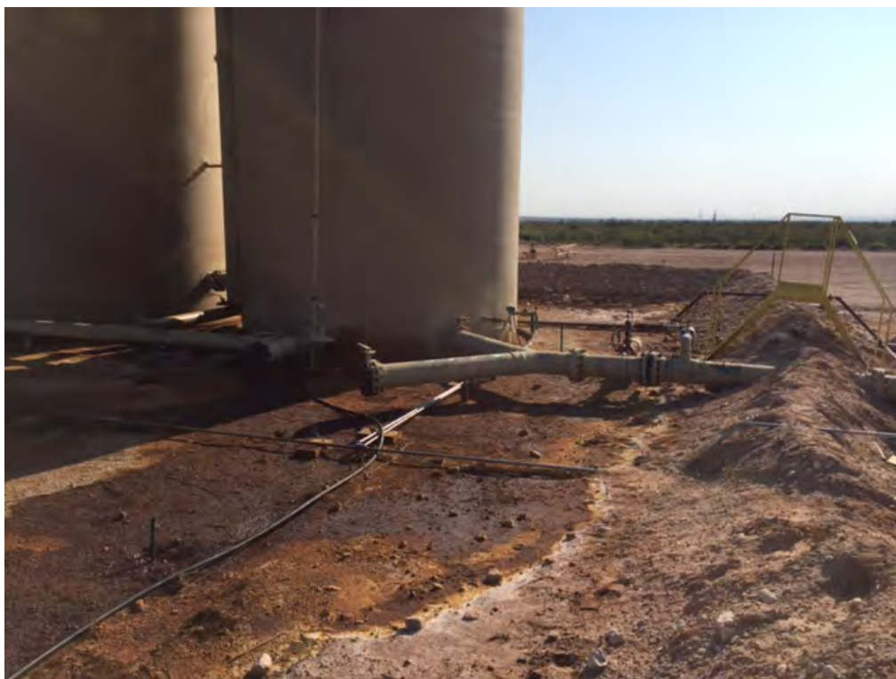
NEL 4 SWD Battery – Release (Looking East-Northeast)
