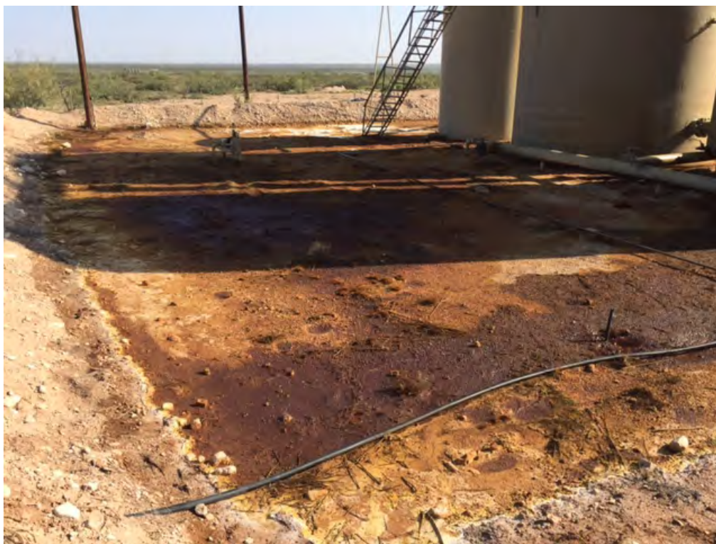
NEL 4 SWD Battery – Release (Looking North-Northeast)
