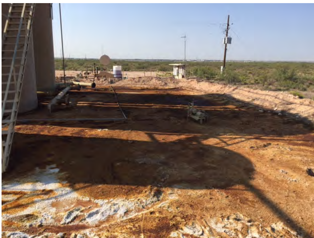
NEL 4 SWD Battery – Release (Looking South)
