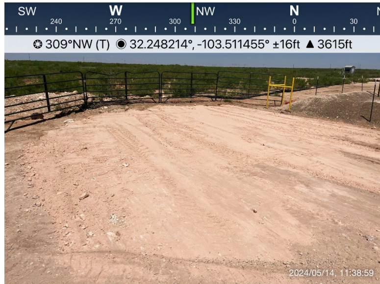
Figure 2: View of the backfilled and restored excavation area.
