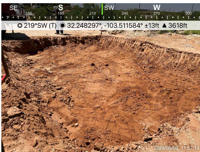
Figure 1: View of final excavation. Date 05/03/2024.
