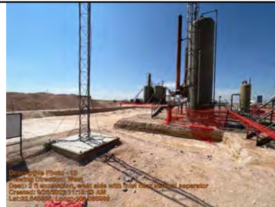
2 ft excavation, west side with inlet near vertical separator
