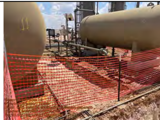
6' deferral excavation between separators
