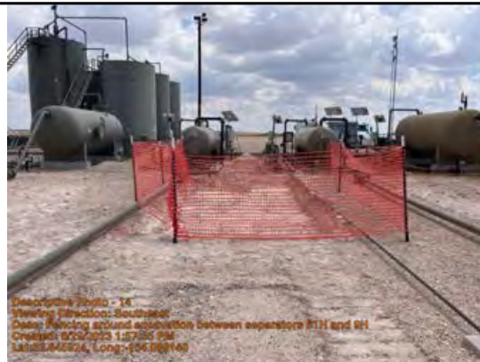
Fencing around excavation between separators 61H and 9H
