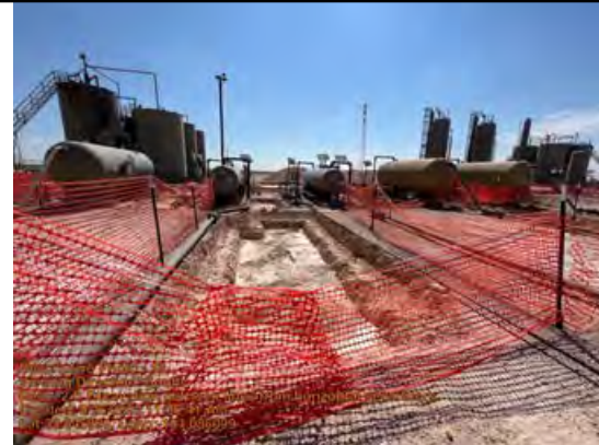
2 ft Excavation between lines from horizontal separators
