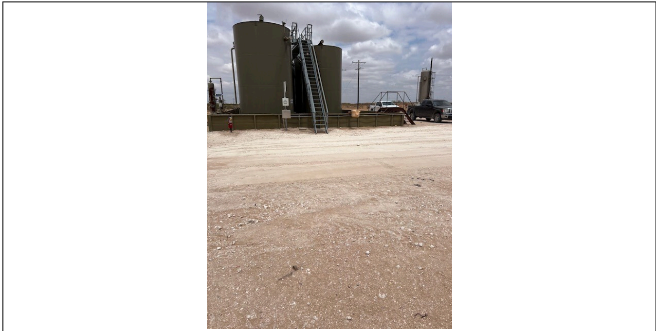
Photograph No. 6 Description: Backfilled area on southeast side of tank battery
