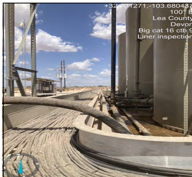
Photo of liner after power washing, taken facing Southeast.
