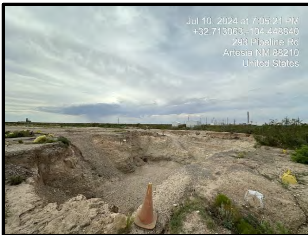
PHOTOGRAPH NO. 7 – A view of the AOC-4/Grid H-5 excavation area upon completion. The view is towards the northeast.
