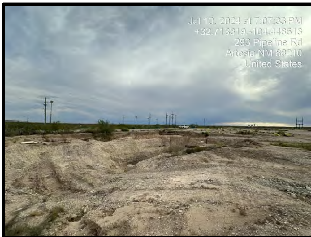
PHOTOGRAPH NO. 8 – An additional view of the AOC-4/Grid H-5 excavation area. The view is towards the southwest.
