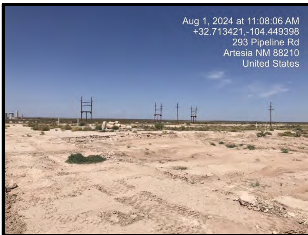
PHOTOGRAPH NO. 11 – A view of the former AOC-7 area treatment cell upon completion of the over-excavation and confirmation sampling activities on August 1, 2024. The view is towards the west.
