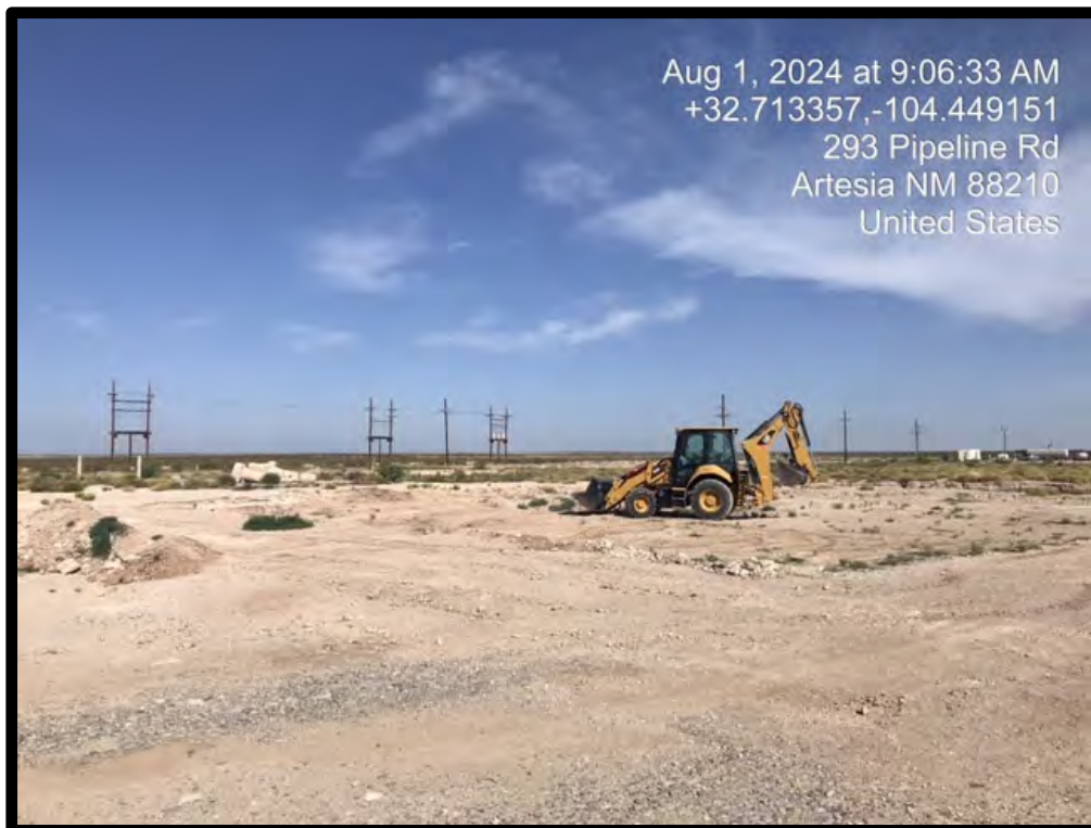
PHOTOGRAPH NO. 11 – A view of the over-excavation activities in the former AOC-7 treatment cell area. The view is towards the west.
