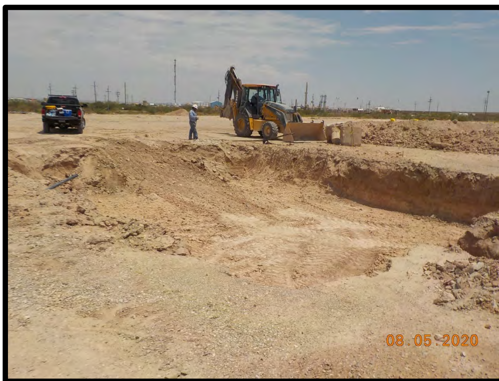
PHOTOGRAPH NO. 3 – A view of the AOC-7 area excavation during the remedial process. The view is towards the southeast.
