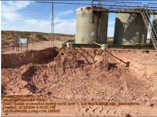
Inside excavation facing north over 1, 2.5, and 3.5 feet bgs excavations.
