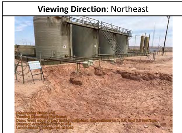
West edge of pad facing northeast. Excavations to 1, 2.5, and 3.5 feet bgs.
