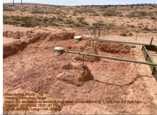
On staircase to tanks facing west. Excavations to 1, 2.5, and 3.5 feet bgs.
