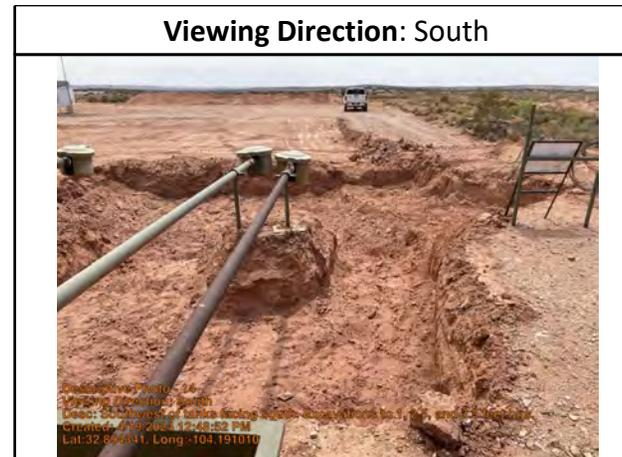
Southwest of tanks facing south. Excavations to 1, 2.5, and 3.5 feet bgs.
