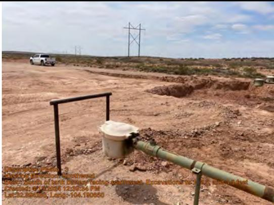
South of tank battery facing southwest. Excavations to 1, 2.5, and 3.5 feet bgs.
