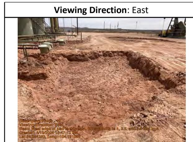
West edge of pad facing east. Excavations to 1, 2.5, and 3.5 feet bgs.
