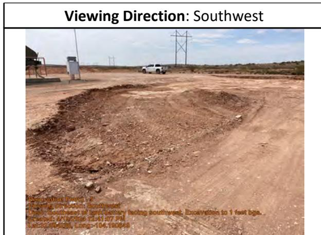
Southeast of tank battery facing southwest. Excavation to 1 feet bgs.
