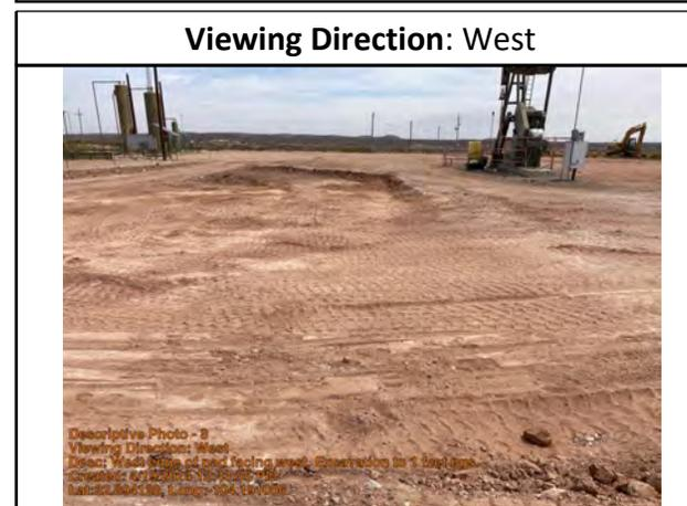
West edge of pad facing west. Excavation to 1 feet bgs.
