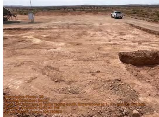
On staircase to tanks facing south. Excavations to 1 and 3.5 feet bgs.
