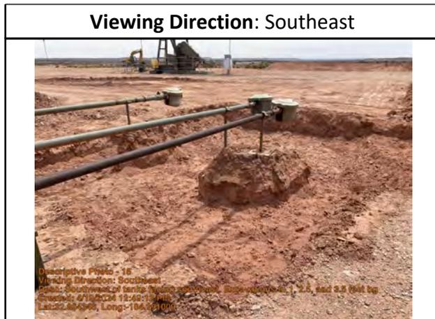
Southwest of tanks facing southeast. Excavations to 1, 2.5, and 3.5 feet bgs.
