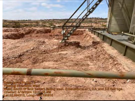
South of tank battery facing west. Excavations to 1, 2.5, and 3.5 feet bgs.
