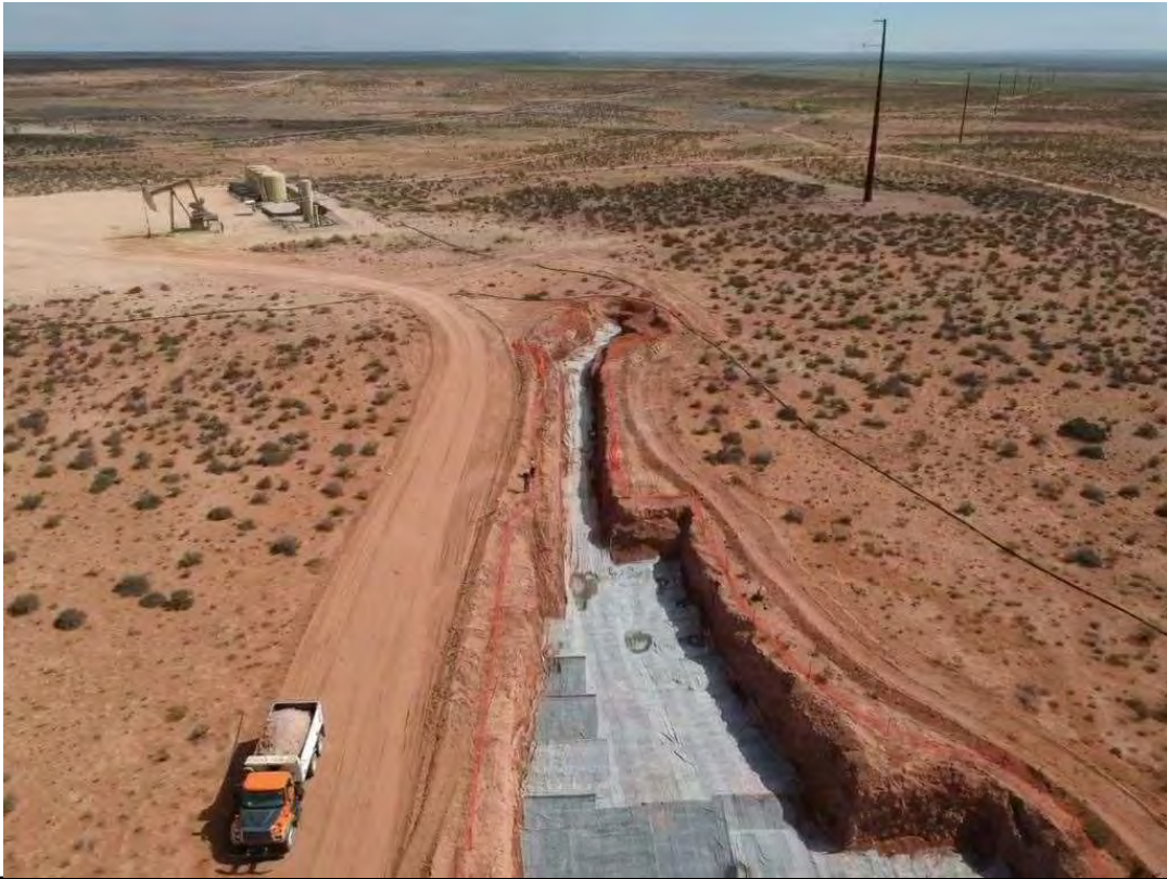
Photo: 25 | Description: Image captured by drone of completed liner installation
