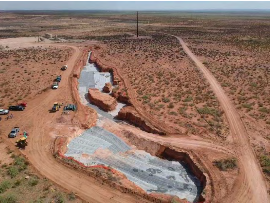
Photo: 26 | Description: Image captured by drone of completed liner installation
