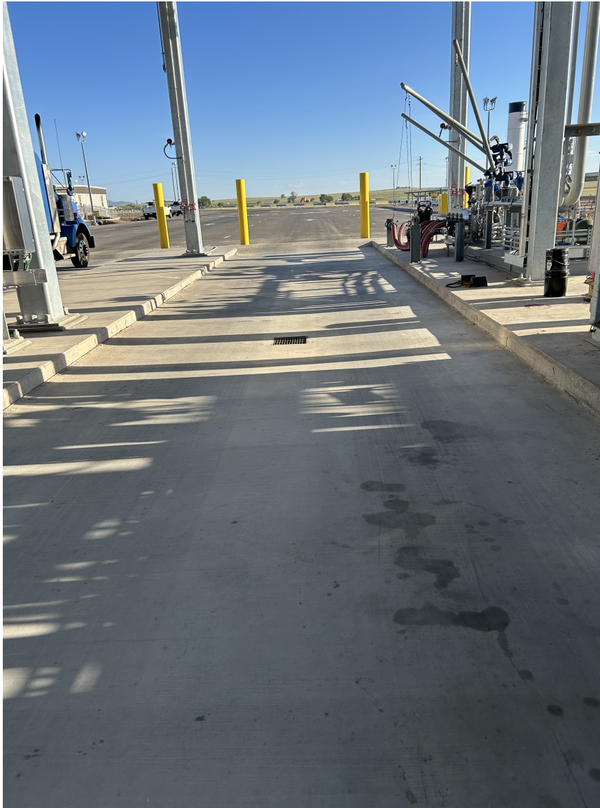
Photo 3: View for the concrete containment after cleaning.
