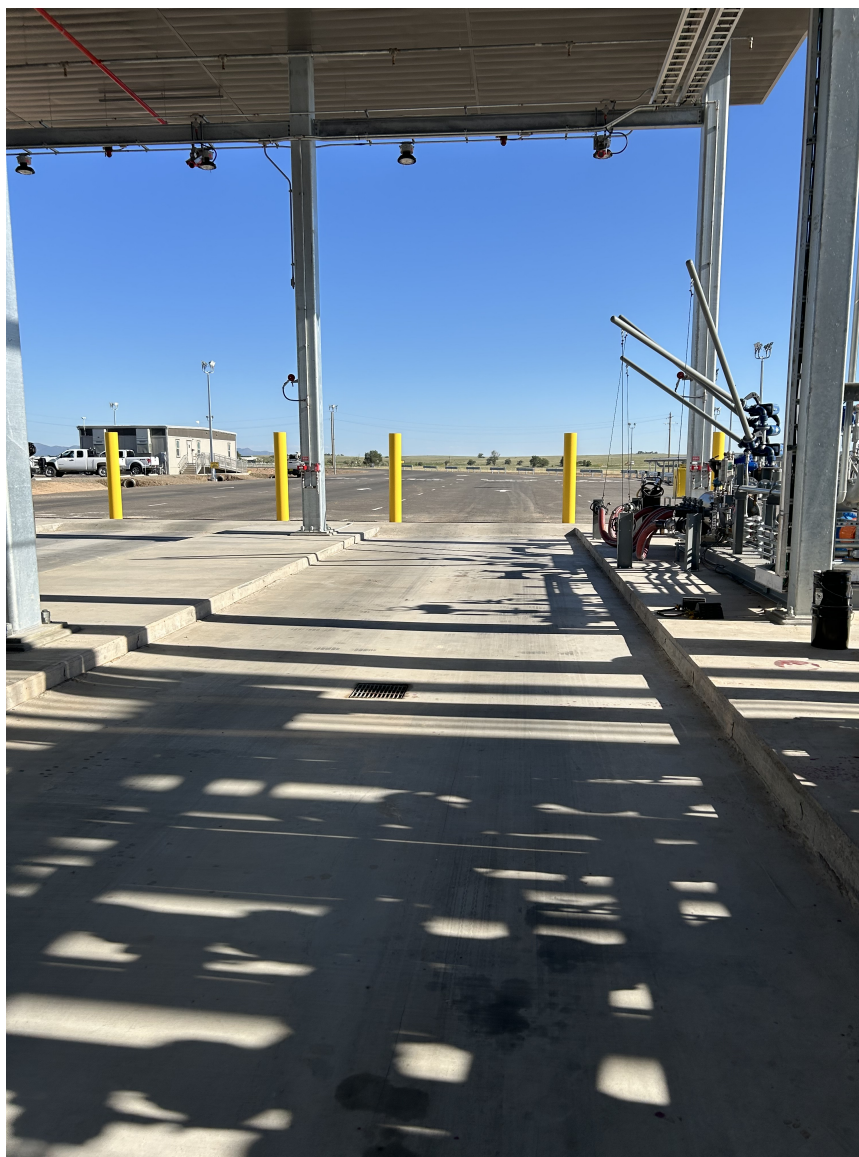
Photo 4: View for the concrete containment after cleaning.
