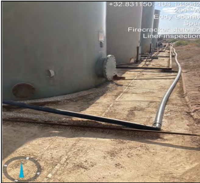
Photo post gravel removal revealing the liner underneath the contaminated gravel facing West
