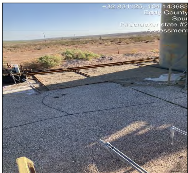
Photograph showing the lined containment area prior to the commencement of gravel removal.
