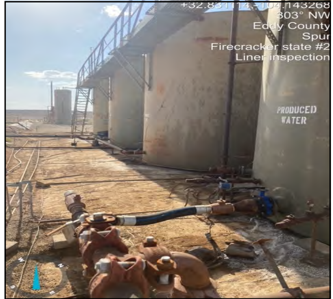
Photo post gravel removal revealing the liner underneath the contaminated gravel facing Northwest
