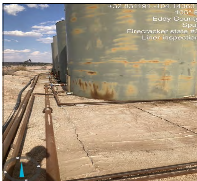
Photo post gravel removal revealing the liner underneath the contaminated gravel facing East.
