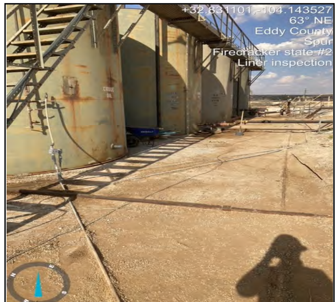
Photo post gravel removal revealing the liner underneath the contaminated gravel facing Northeast
