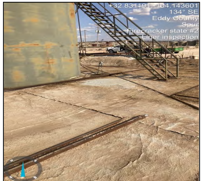
Photo post gravel removal revealing the liner underneath the contaminated gravel facing Southeast
