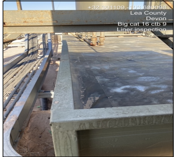
Photograph depicting the condition of the liner following the extraction of produced water by a vacuum truck, oriented facing.
