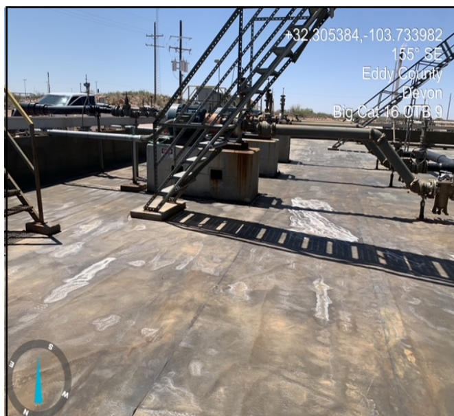
Photograph depicting the condition of the liner following the extraction of produced water by a vacuum truck, oriented facing Southeast.
