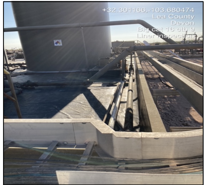
Photograph depicting the condition of the liner following the extraction of produced water by a vacuum truck.
