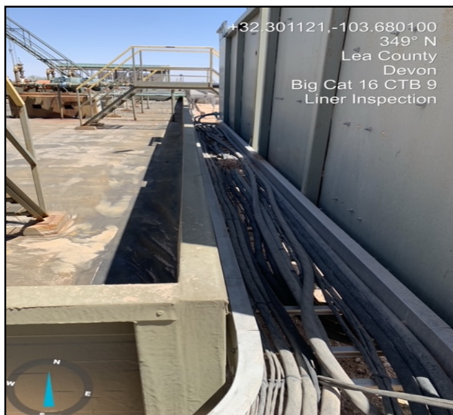
Photograph depicting the condition of the liner following the extraction of produced water by a vacuum truck, oriented facing North.
