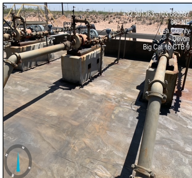
Photograph depicting the condition of the liner following the extraction of produced water by a vacuum truck, oriented facing Northeast.
