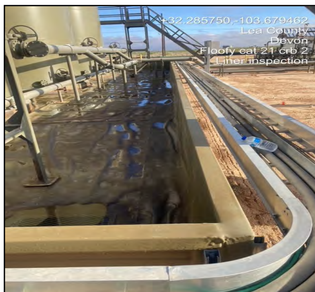
Photograph depicting the condition of the liner.
