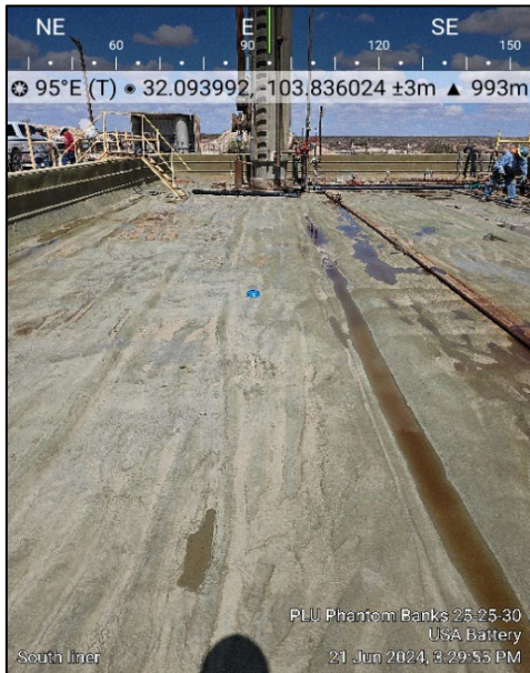
Photograph: 3 Date: 6/21/2024 Description: Liner post vacuum truck activities. View: East
