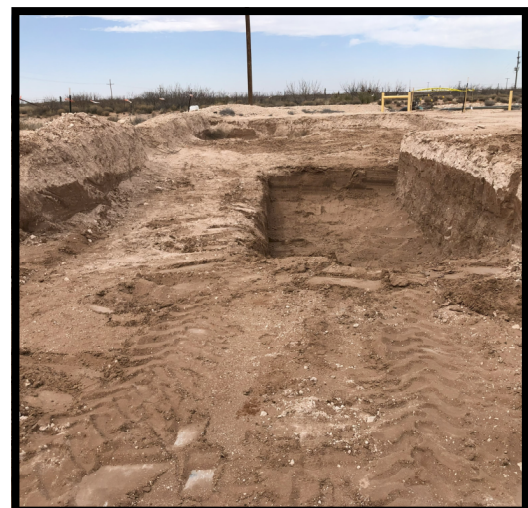
Area requiring additional excavation to greater depth (SW 91H-Bottom 8)
