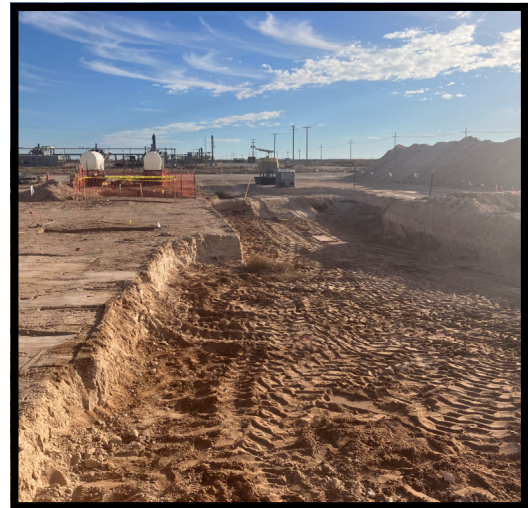
View of excavation, facing south
