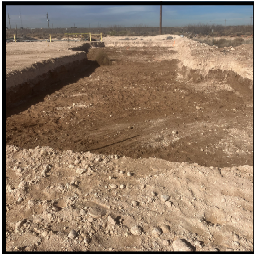
View of excavation, facing north
