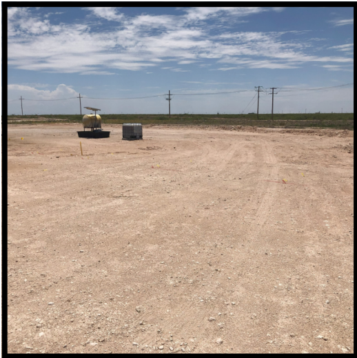
View of backfilled excavation, facing southwest
