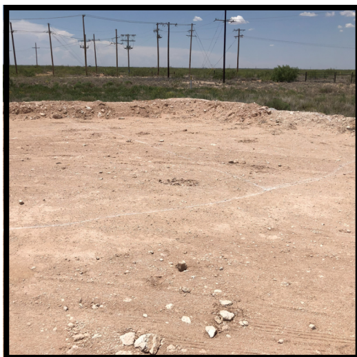
View of backfilled excavation, facing northwest
