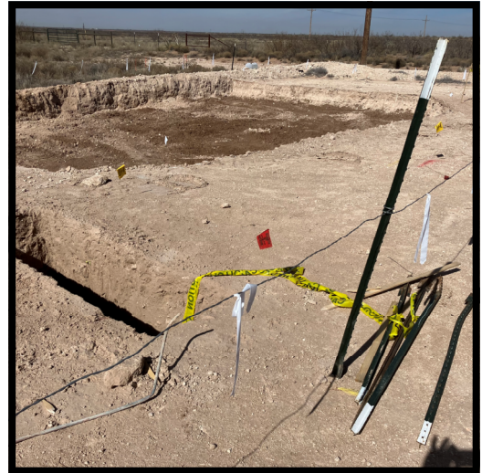
Location of gas line on eastern edge of excavation area
