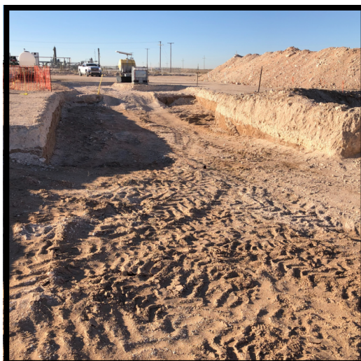
View of excavation, facing south
