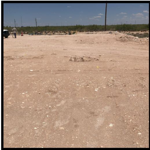
View of backfilled excavation, facing north
