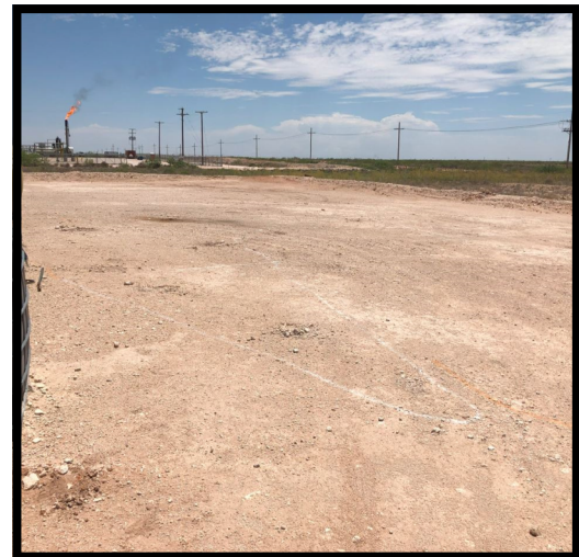
View of backfilled excavation, facing southwest
