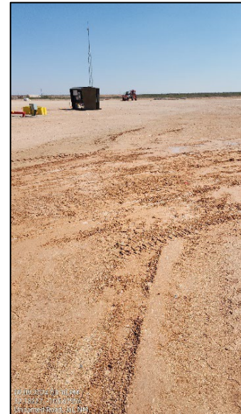
Photograph: 4 Date: 9/9/2024 Description: Backfilled excavation View: South
