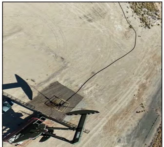
Aerial Photo of the site post-assessment, showcasing the current layout and condition.
