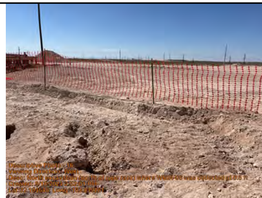
Viewing Direction: West
