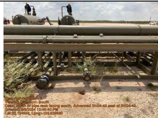
Viewing Direction: South
