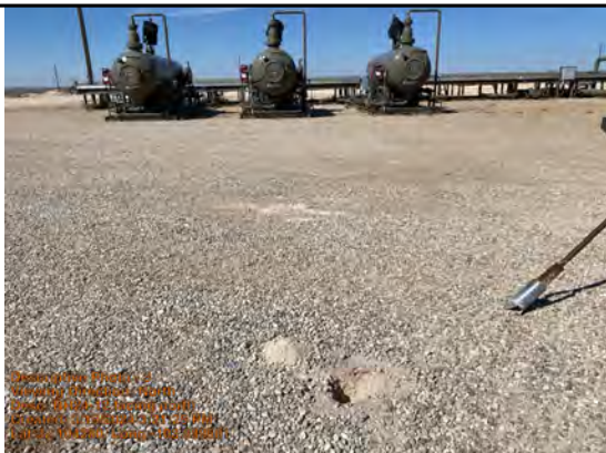
BH24-12 facing north
