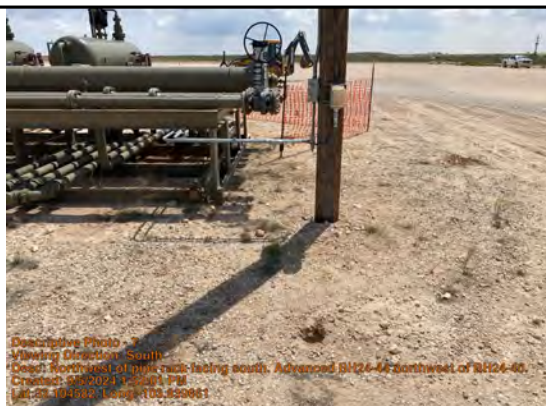
Viewing Direction: South
