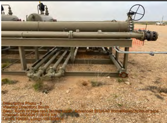
Viewing Direction: South
