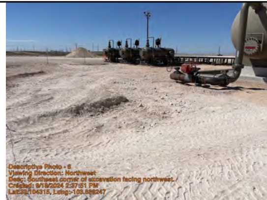
Southeast corner of excavation facing northwest.
