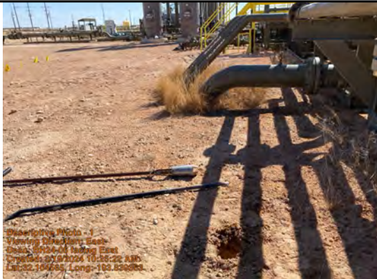
BH24-06 facing East
