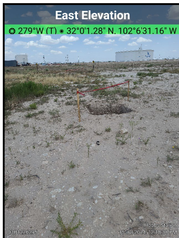
View of historical release extent after hydro-excavation delineation activities, facing west (07/15/24).
