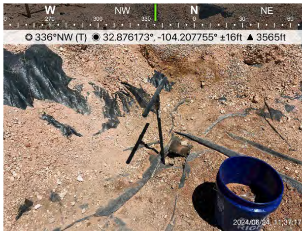
Figure 6. Hole in the liner (CS-03)
