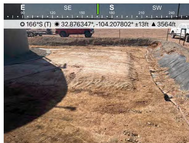
Figure 9. Soil conditions after liner removal.
