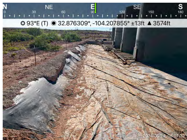
Figure 1. Initial Liner Inspection.
