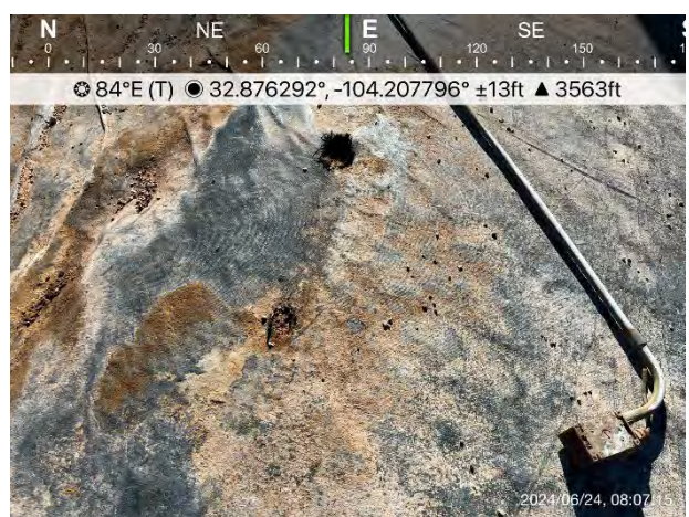
Figure 5. Hole in the liner (CS-02)
