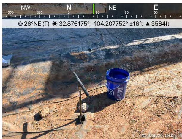
Figure 4. Hole in the liner (CS-01)
