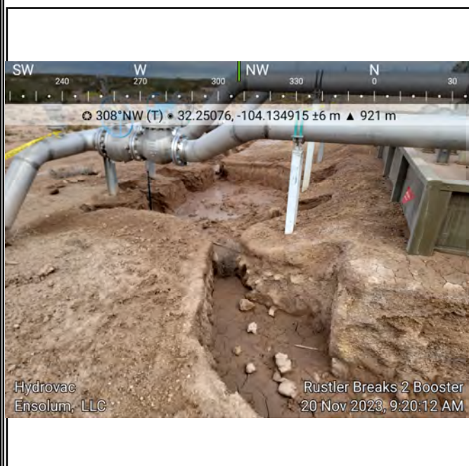
Photograph 15 Date: 11/20/2023 Description: Hydrovac Containment View: Northwest
