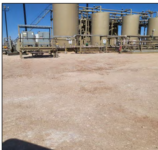
Photograph: 7 Date: 8/8/2023 Description: Backfilled excavation on pad View: North
