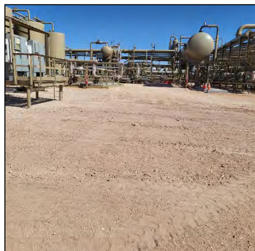
Photograph: 6 Date: 8/8/2023 Description: Backfilled excavation on pad View: East
