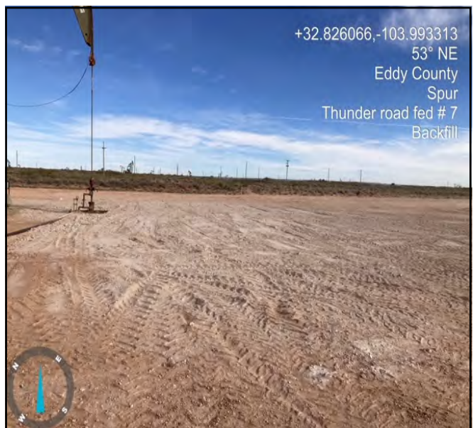
Photo of the excavated area backfilled with clean material facing Northeast.
