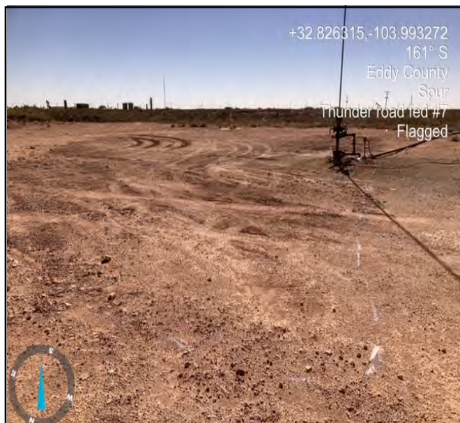
Site being flagged for excavation by site tech facing South.
