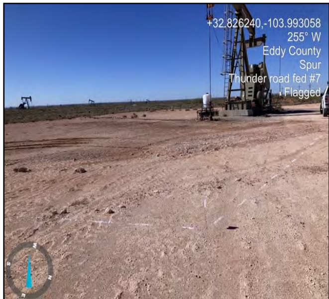
Site being flagged for excavation by site tech facing West.
