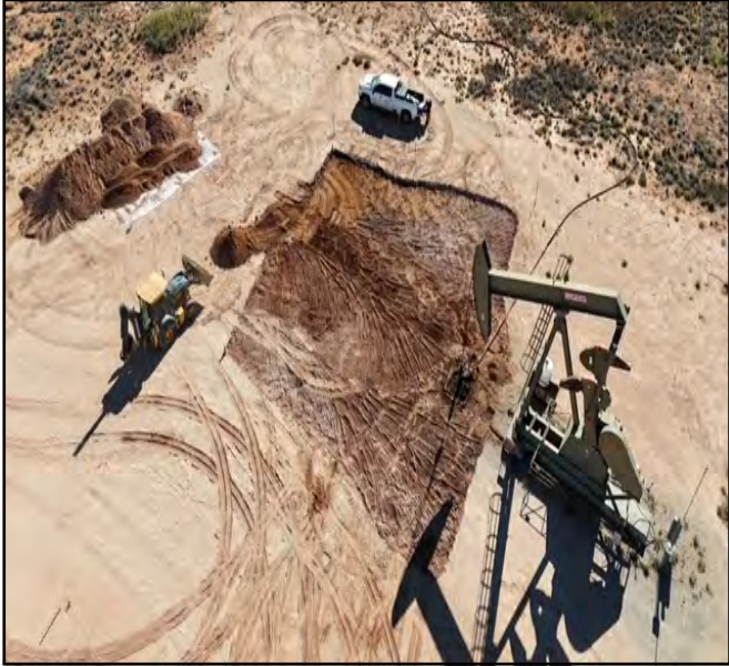
Photo of the flagged area excavated completely, photo taken by drone.
