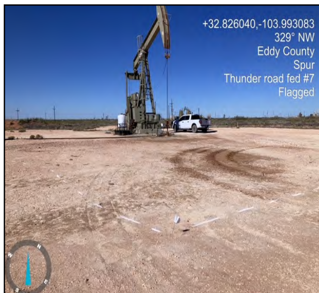
Site being flagged for excavation by site tech facing Northwest.
