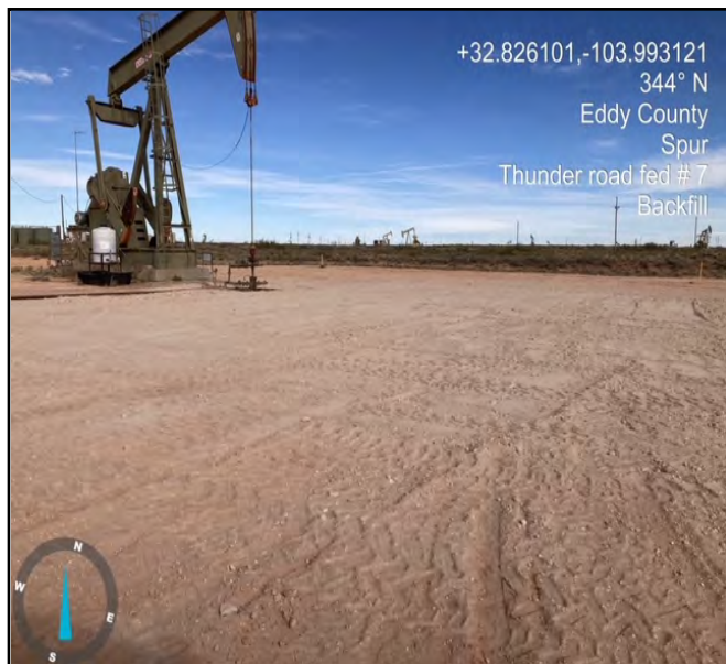
Photo of the excavated area backfilled with clean material facing North.
