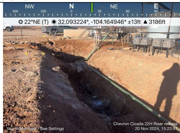
Photo 6: nAPP2424378052 piping repair excavation area.
