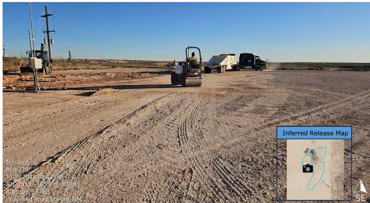
Excavation Area Being Backfilled and Compacted
