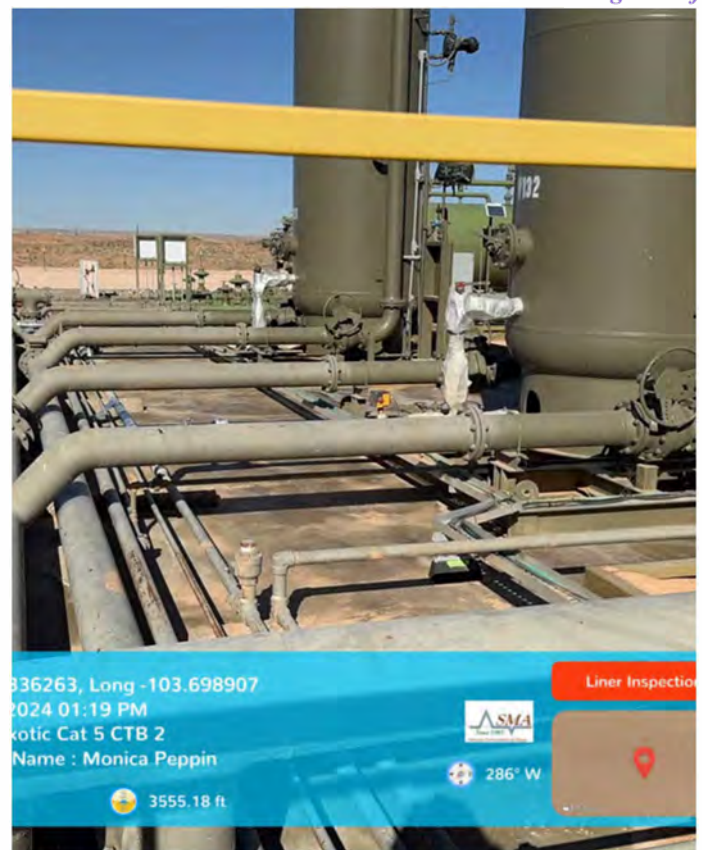
Photograph #19: Liner under piping and equipment in northeast corner
