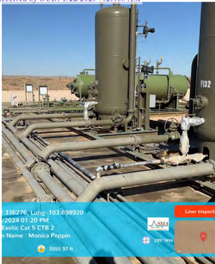
Photograph #22: View of liner around heater treaters and under piping
