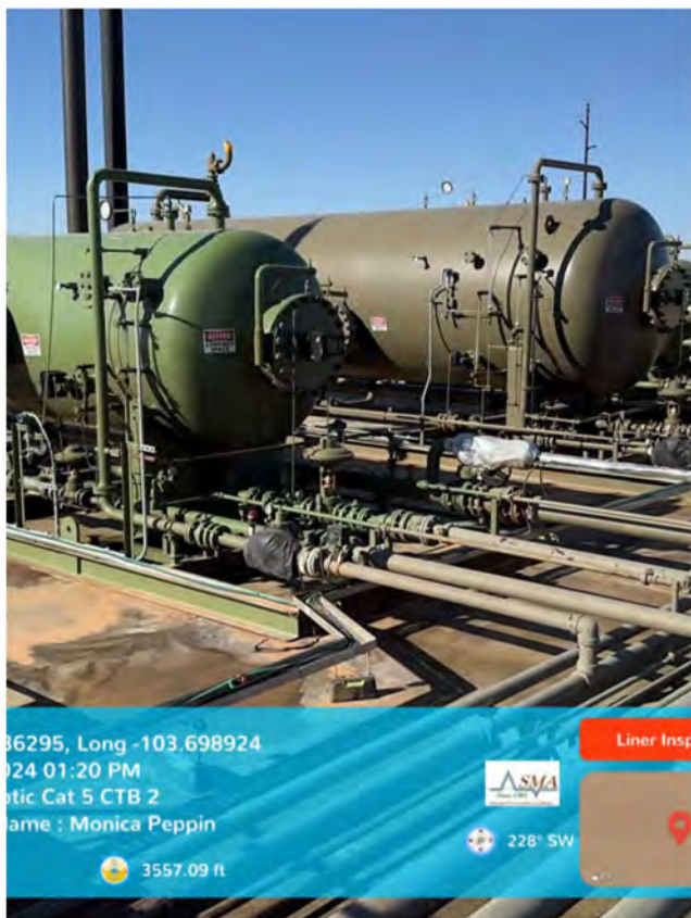
Photograph #24: View of liner underneath piping
