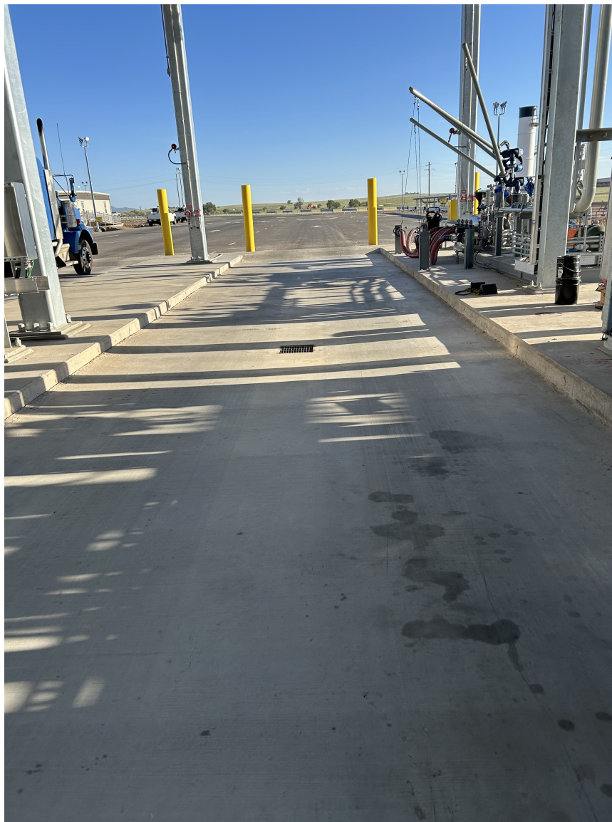
Photo 3: View for the concrete containment after cleaning.
