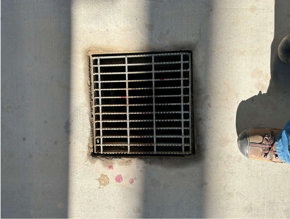
Photo 5: View for the concrete containment drain to the sump.
