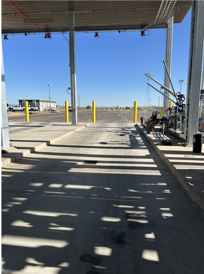
Photo 4: View for the concrete containment after cleaning.
