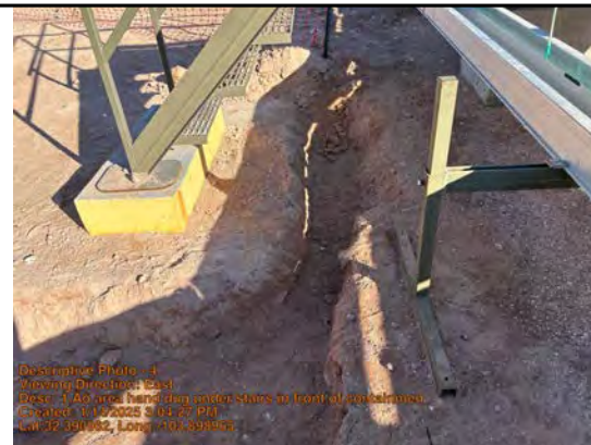
1' area hand dug under stairs in front of containment
