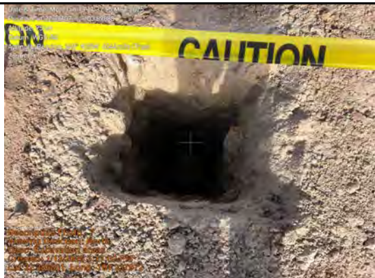
areas hydro vac to window out electrical lines
