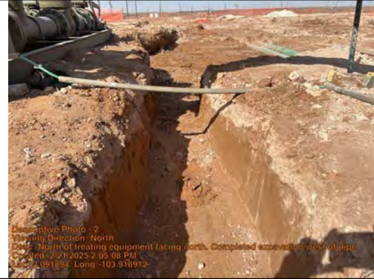
North of treating equipment facing north. Completed excavation west of pipelines to 2 feet bgs.
