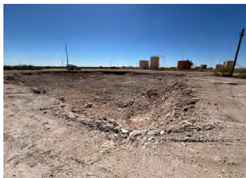
View to W of excavation (9/25/24).
