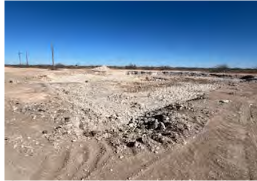
View to NE of excavation (1/15/25).
