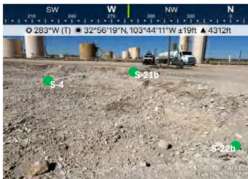
View to W of excavation with sample points (2/25/25).
