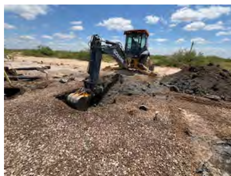
View of initial investigation (6/10/24).
