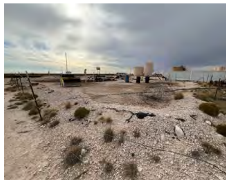
View of staining in bermed area to east of well pad (11/27/23)
