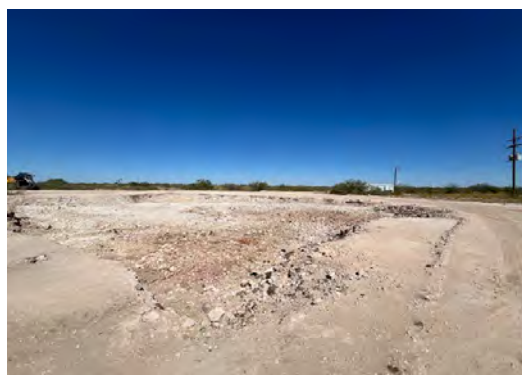
View to E of excavation (9/25/24).
