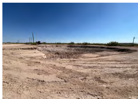
View to N of excavation at former pump area (8/28/24).
