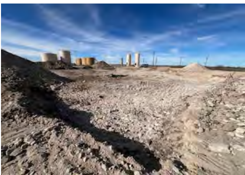
View to SW of excavation (12/26/25).
