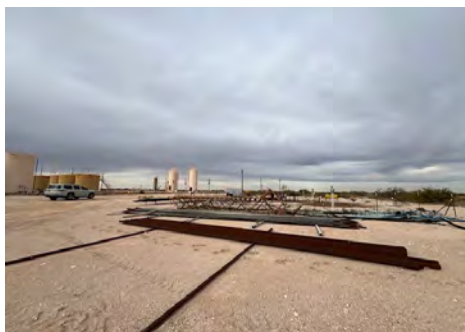
View of area at west side of TB (11/27/23).
