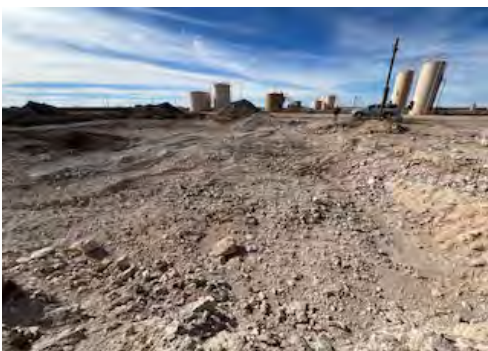
View to W of excavation (12/26/25).
