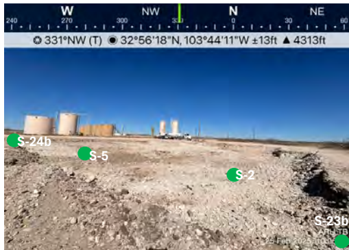
View to NW of excavation with sample points (2/25/25).
