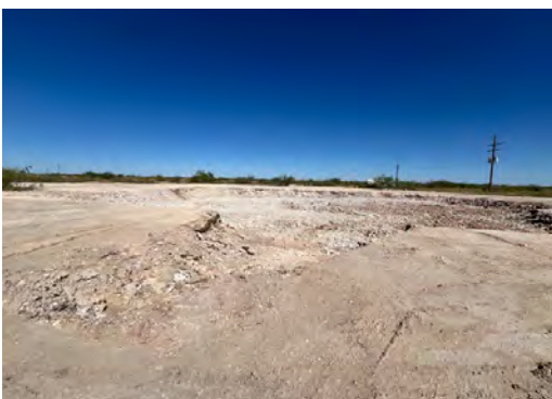
View to E of excavation (9/25/24).
