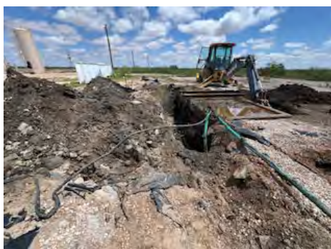
View of initial investigation (6/10/24).
