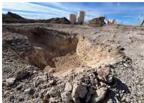
View to NW of excavation (12/26/25).
