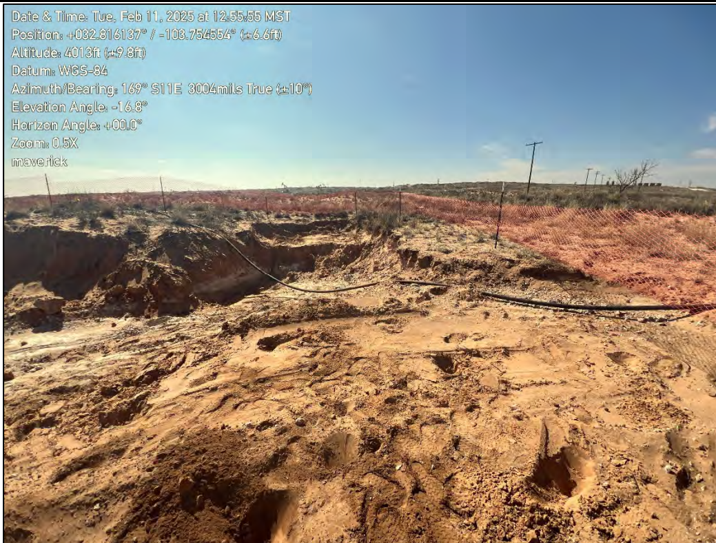
PHOTO 5: Southeastern view of excavation extent. 02/11/2025
