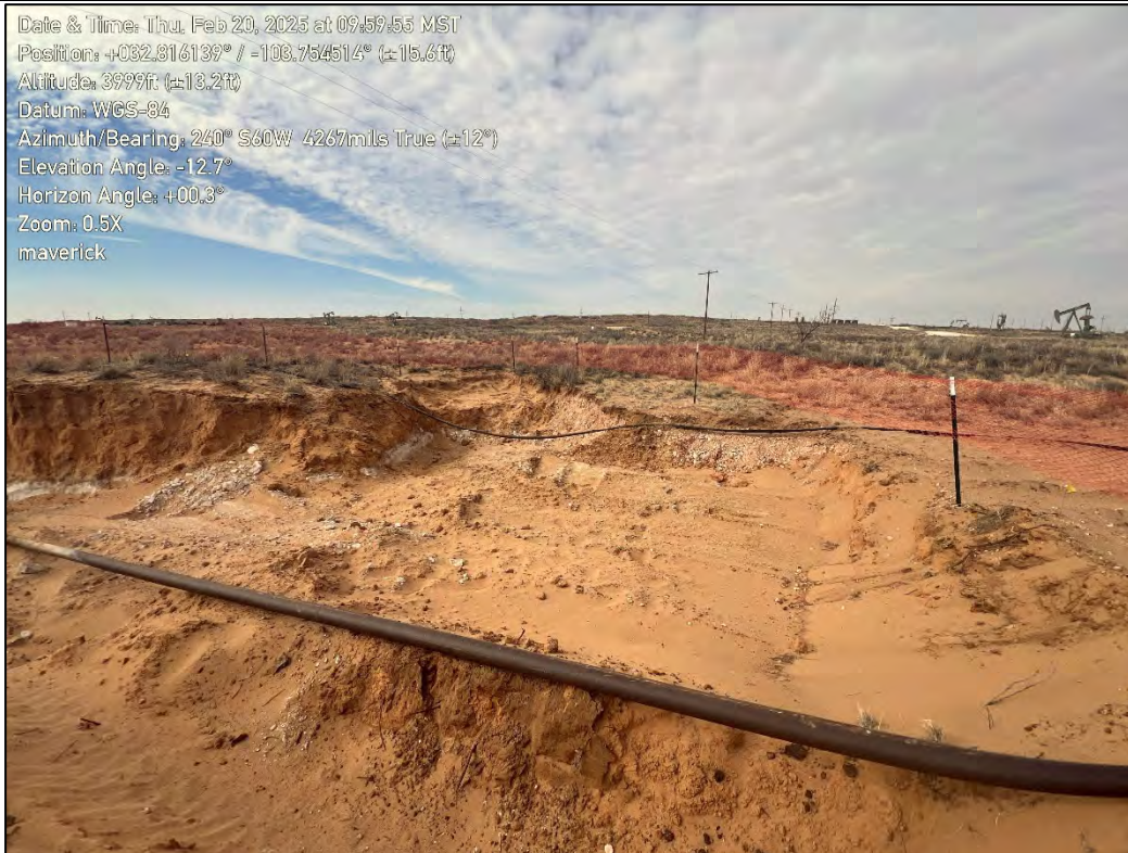
PHOTO 7: Southwestern view of excavation extent. 02/20/2025
