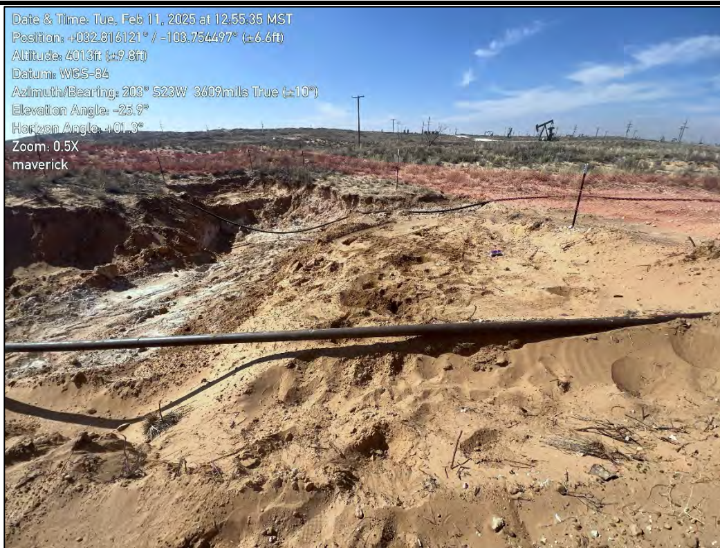
PHOTO 4: Southwestern view of excavation extent. 02/11/2025
