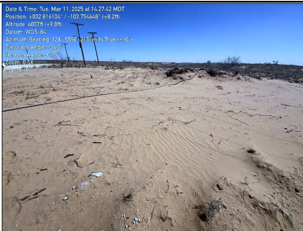
PHOTO 10: Southeastern view after restoration activities. 03/11/2025
