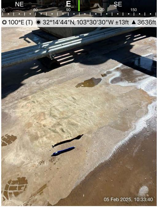
Figure 2: Edge of previous patch lifted; no penetration of barrier
