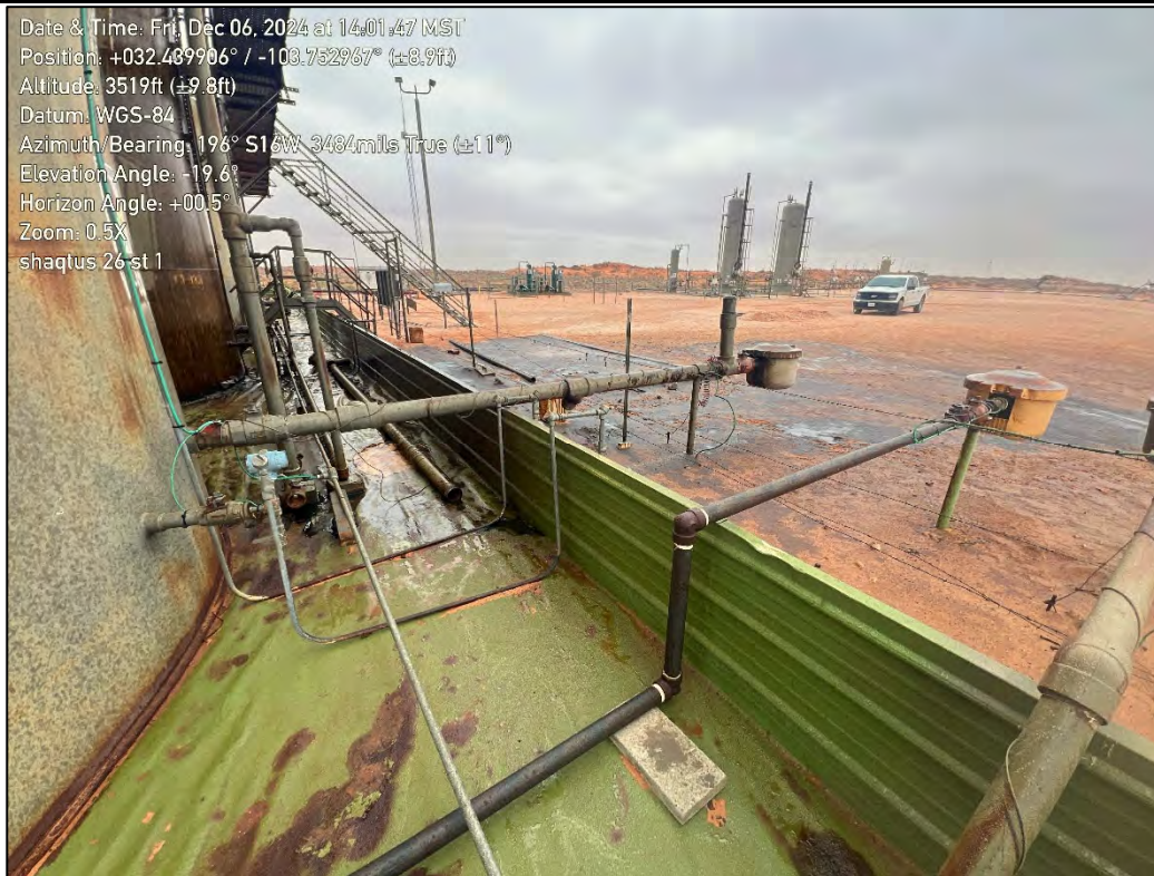
PHOTO 1: Southwestern view during initial site assessment activities. 12/6/2024
