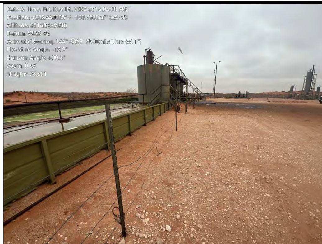
PHOTO 2: Southeastern view during initial site assessment activities. 12/6/2024
