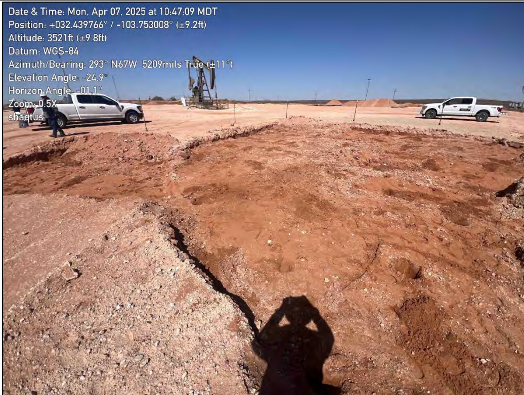
PHOTO 21: Northwestern view of excavation extent. 4/7/2025
