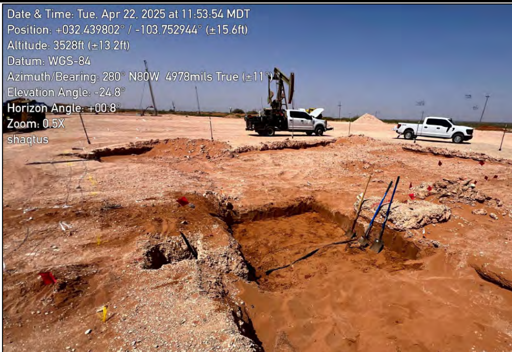
PHOTO 22: Northwestern view of excavation extent. 4/22/2025
