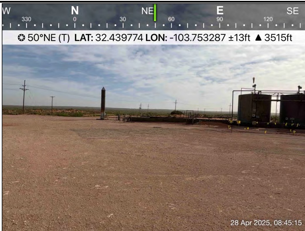
PHOTO 24: Northeastern view after restoration activities. 4/28/2025
