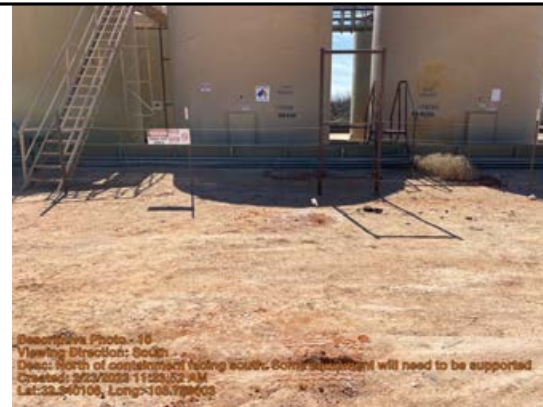
North of containment facing south. Some equipment will need to be supported, diverted, or moved during excavation.
