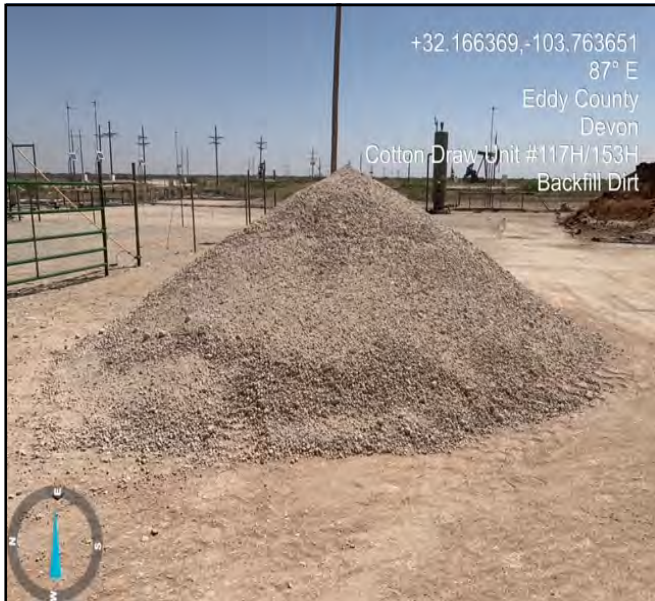
Photograph of clean backfill material facing east.
