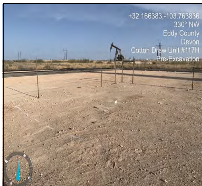
Photograph of site tech showing location prior to excavation, facing northwest.
