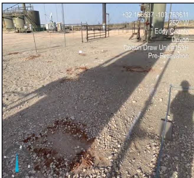
Photograph of site tech showing location prior to excavation facing west.
