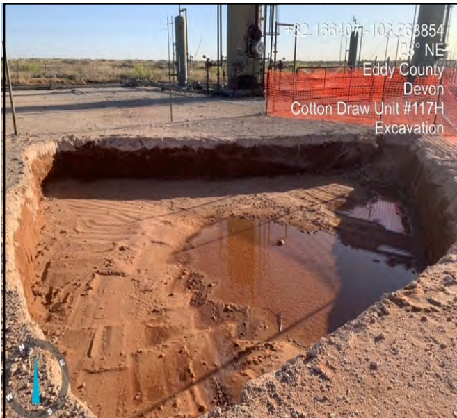
Photograph taken during excavation facing northeast.
