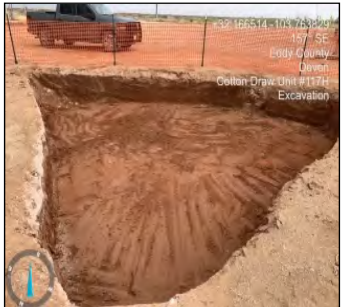
Photograph taken during excavation facing southeast.
