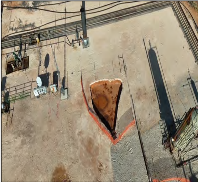
Photograph taken during excavation
