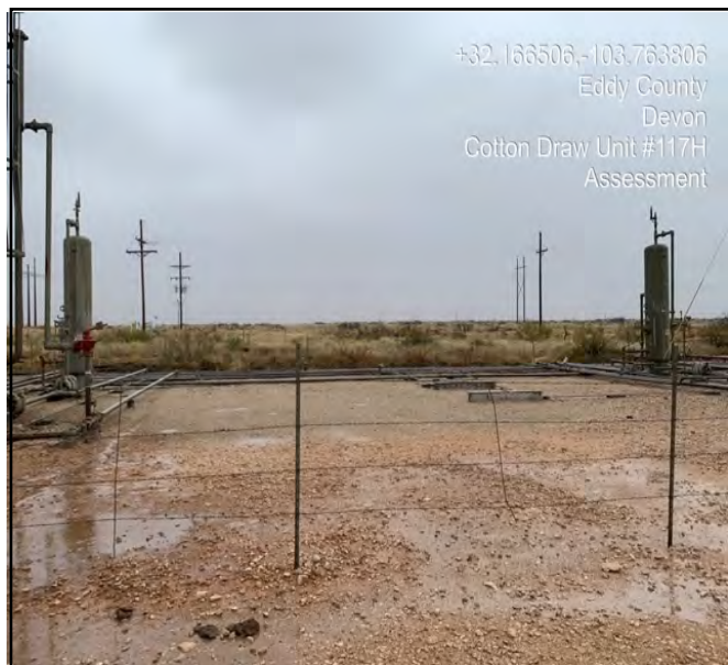
Photograph taken during site assessment
