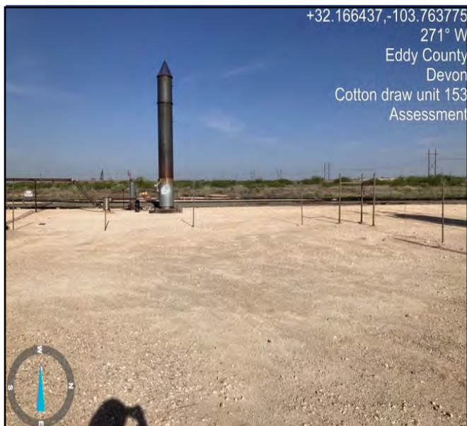
Photograph taken during assessment facing west.
