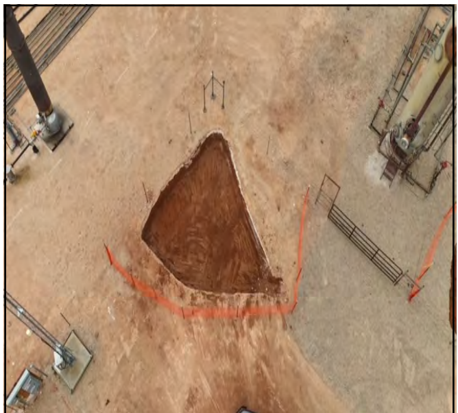
Photograph taken during excavation.
