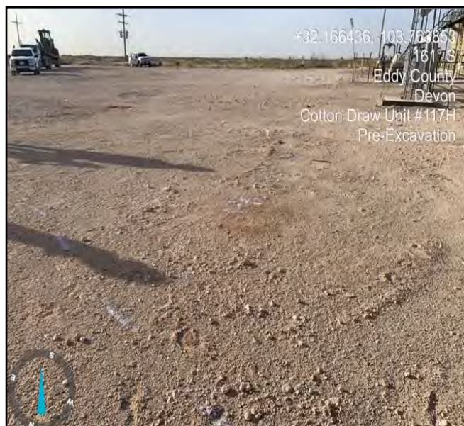
Photograph of site tech showing location prior to excavation, facing south.
