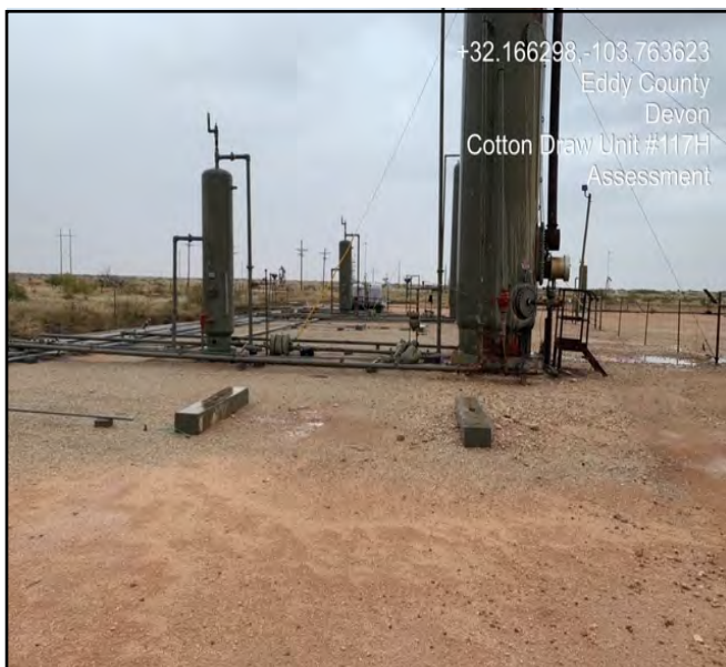
Photograph taken during site assessment
