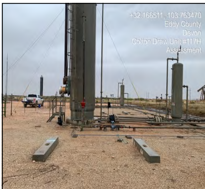
Photograph taken during site assessment
