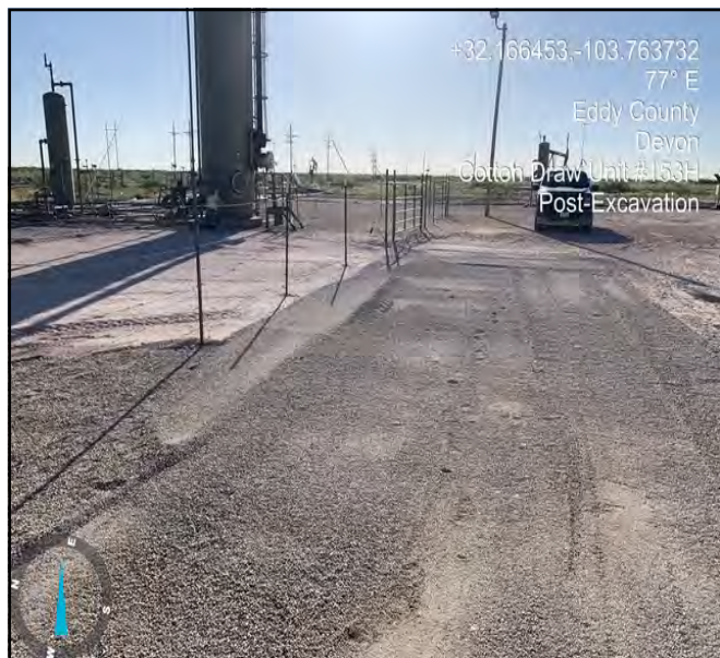
Photo taken post excavation facing east.
