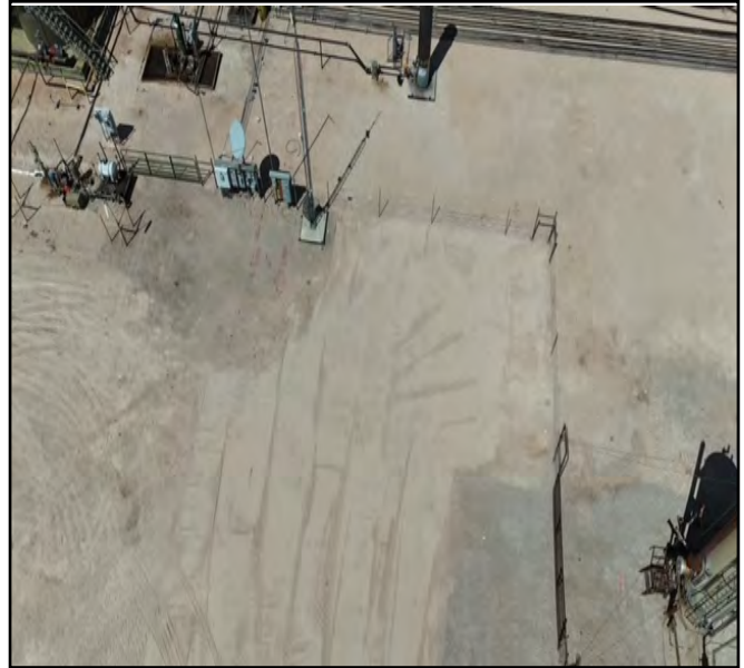
Photo taken post excavation
