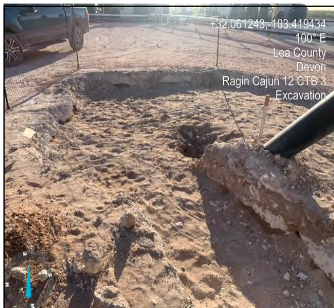
Pictures taken during excavation, Facing East.
