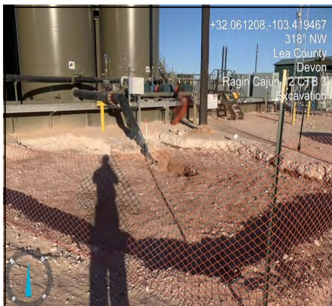
Pictures taken during excavation, Facing Northwest.
