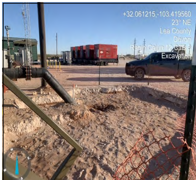
Pictures taken during excavation, Facing Northeast.
