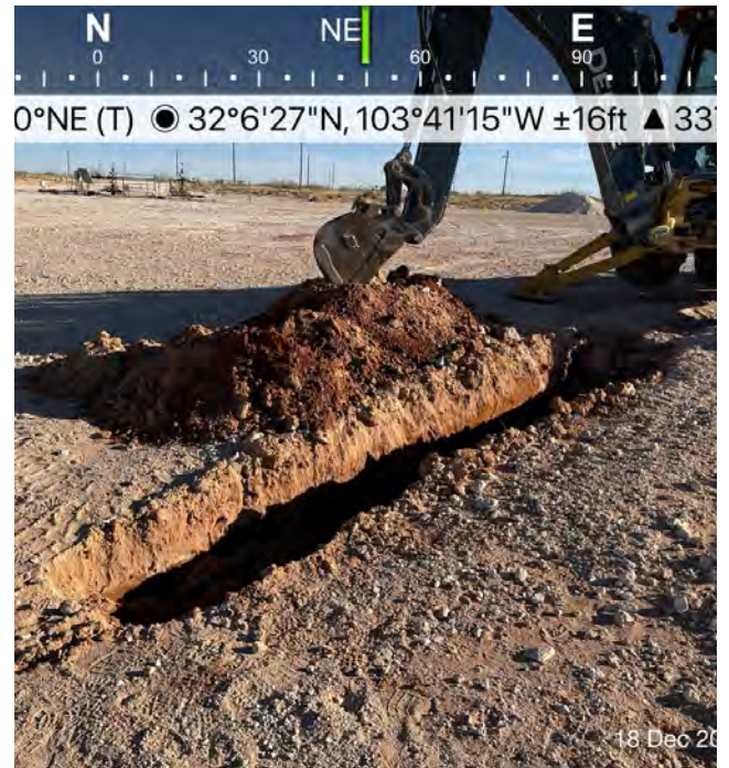
View of equipment being utilized to pothole for sample collection
