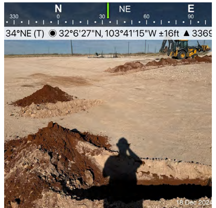
Test pit trenched for multiple samples to be collected
