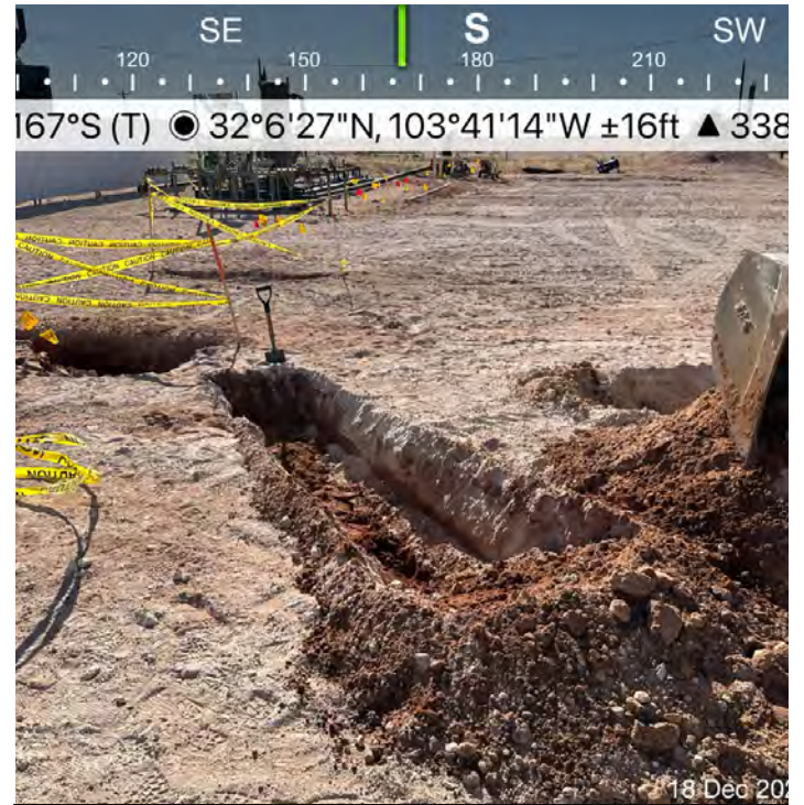
Test pit trenched for multiple samples to be collected
