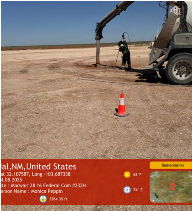
Facing northwest viewing crew daylighting lines within area of excavation
