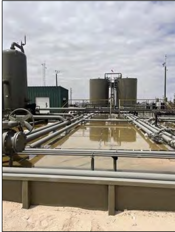
PHOTO 1: Western view during initial site assessment by WPX. 4/17/2025
