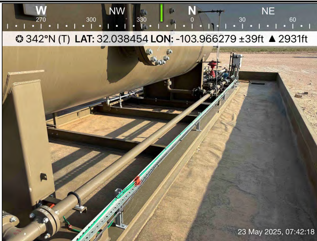
PHOTO 19: Northwestern view during liner inspection activities. 5/23/2025
