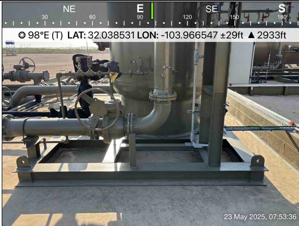
PHOTO 17: Southeastern view during liner inspection activities. 5/23/2025
