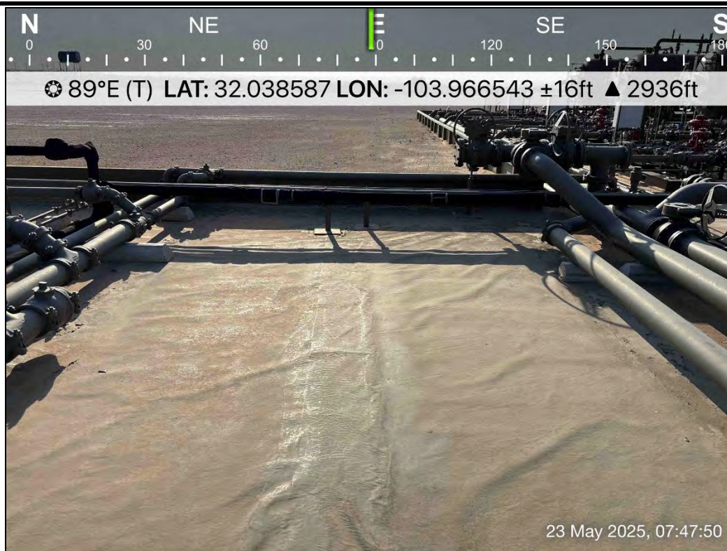
PHOTO 11: Eastern view during liner inspection activities. 5/23/2025
