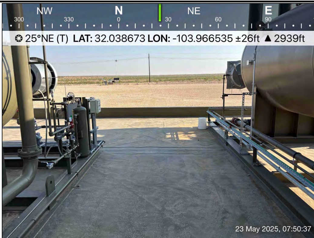
PHOTO 13: Northeastern view during liner inspection activities. 5/23/2025
