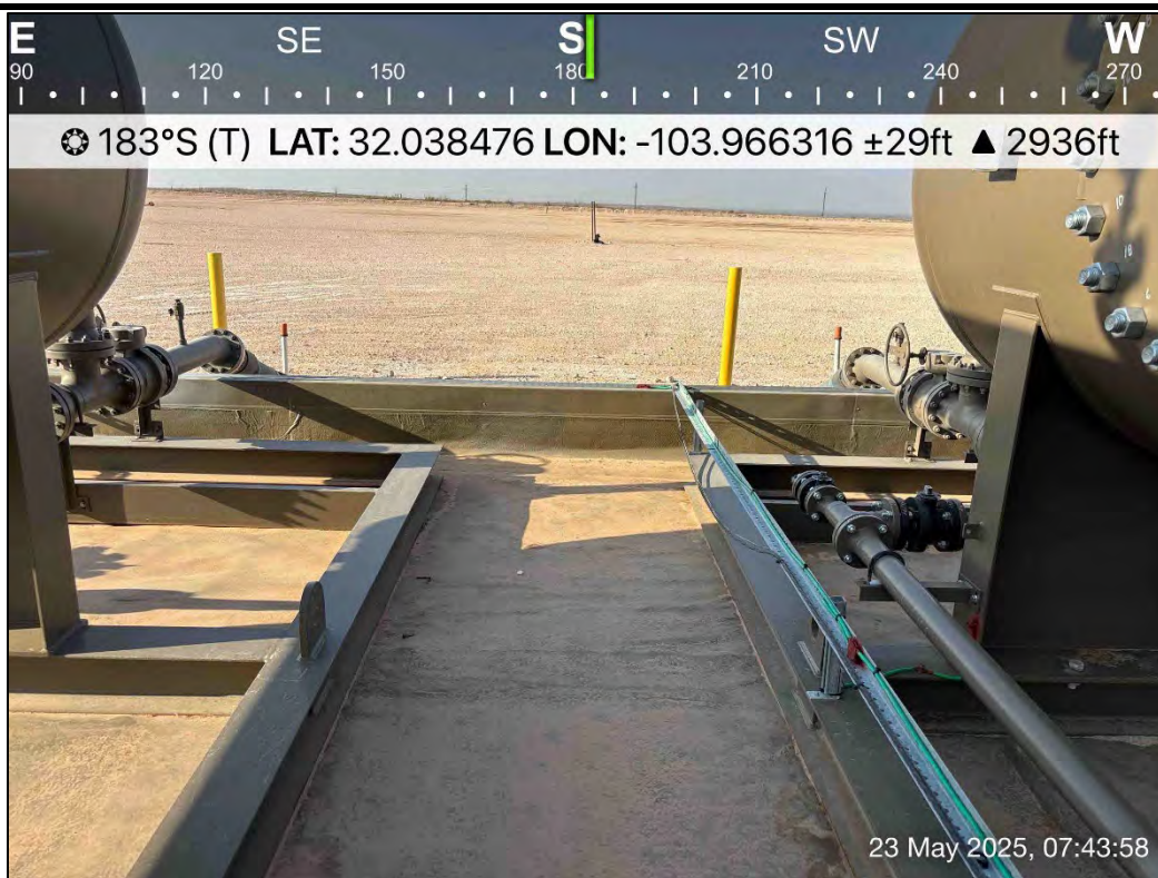
PHOTO 20: Southern view during liner inspection activities. 5/23/2025
