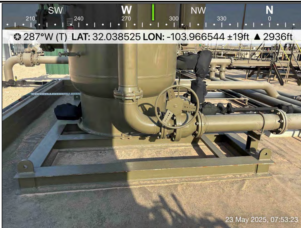
PHOTO 16: Northwestern view during liner inspection activities. 5/23/2025
