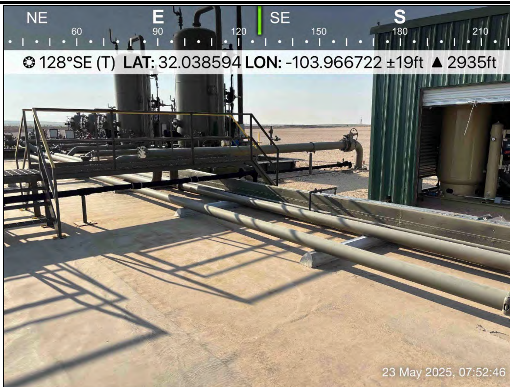
PHOTO 15: Southeastern view during liner inspection activities. 5/23/2025
