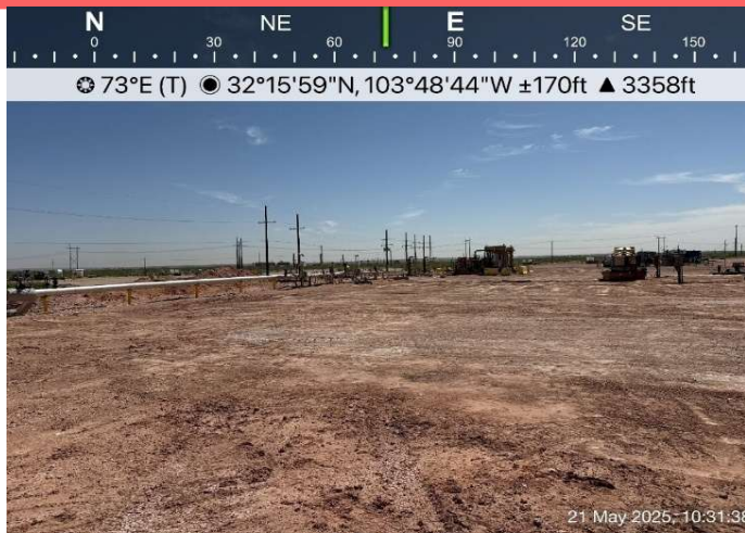
View of Area of Concern
