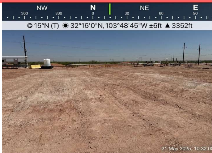
View of Area of Concern
