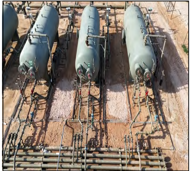
Aerial photo of the site backfilled with clean material.
