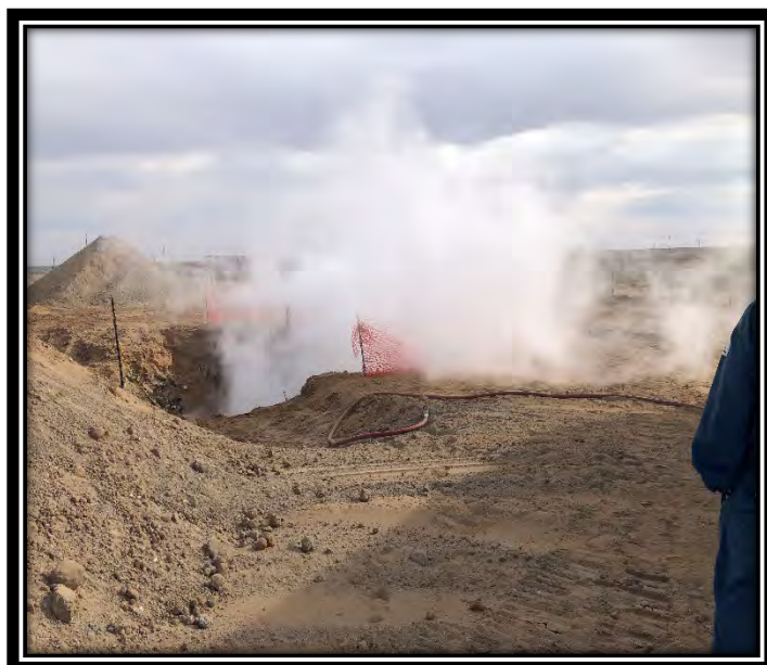
Picture 6: Hydrogen Peroxide Application (View 4)
