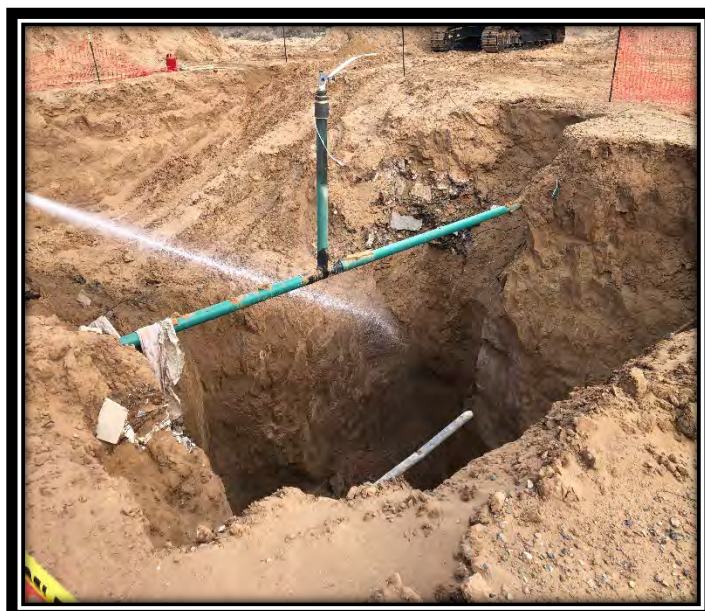
Picture 4: Hydrogen Peroxide Application (View 2)
