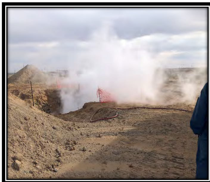
Picture 6: Hydrogen Peroxide Application (View 4)
