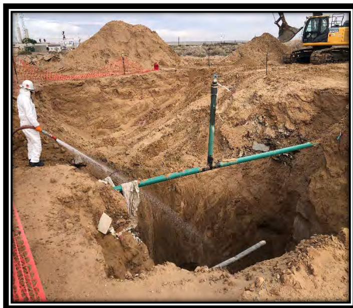
Picture 3: Hydrogen Peroxide Application (View 1)
