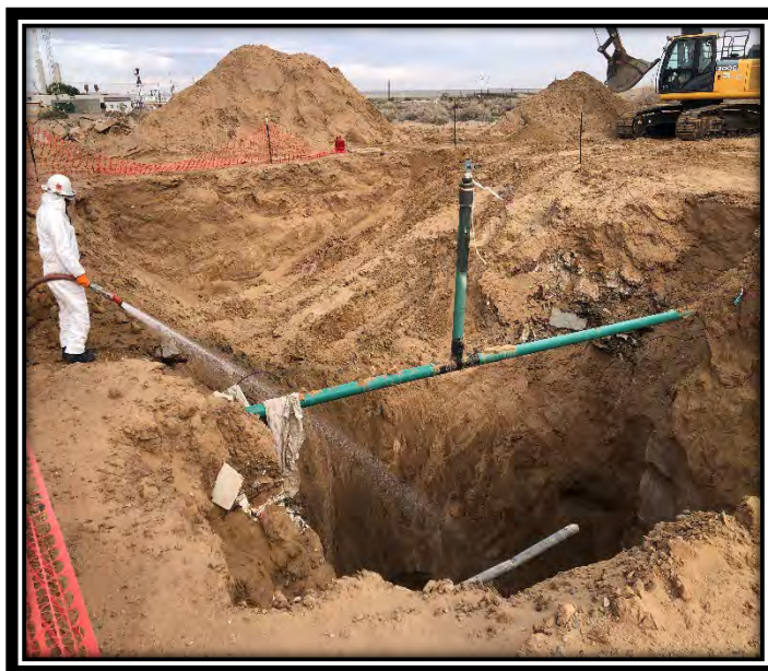
Picture 3: Hydrogen Peroxide Application (View 1)
