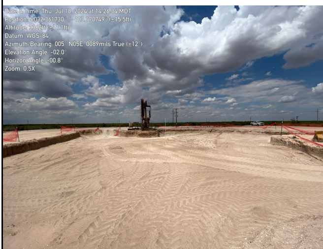
Photograph: 4 Date: 7/18/2024 Description: Excavation Activities View: North
