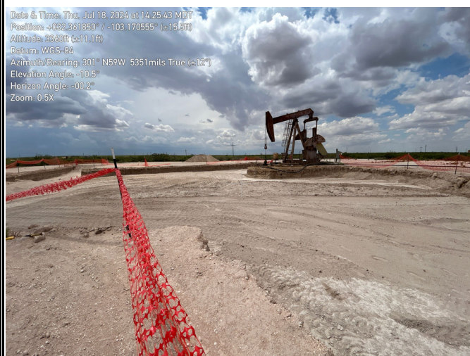
Photograph: 3 Date: 7/18/2024 Description: Excavation activities View: Northwest
