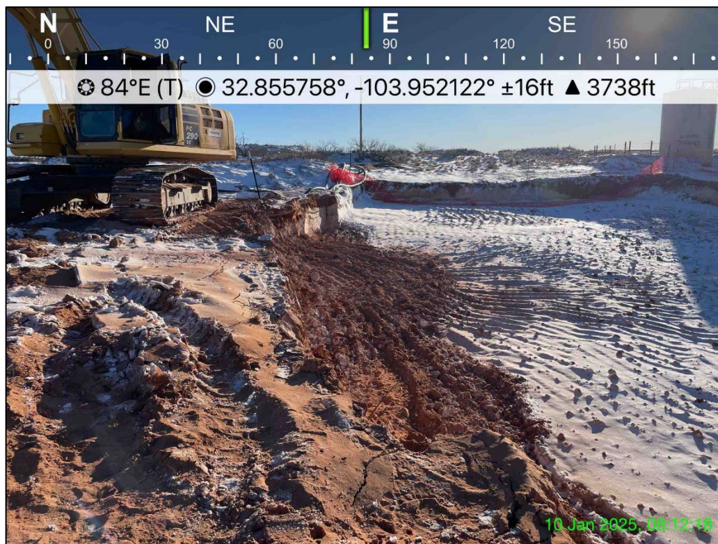
Photo 3: ~1 foot of topsoil observed in northeast corner of excavation, facing northeast
