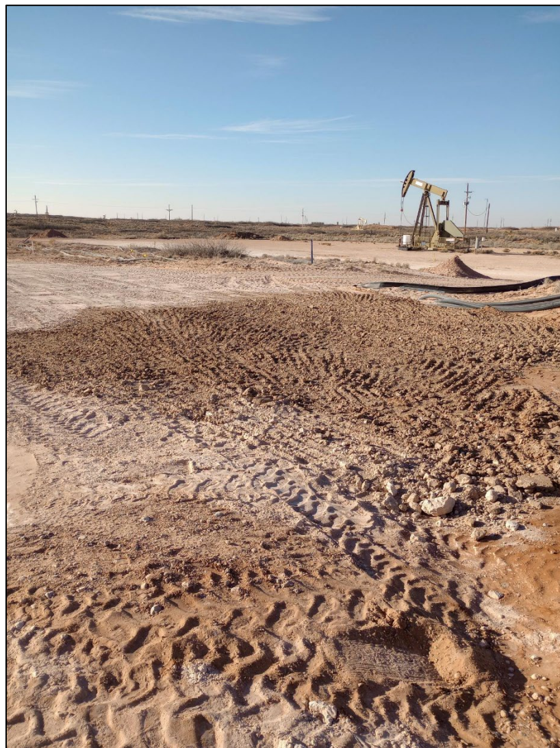
Photo 10: Area backfilled with topsoil, seeded with BLM #2 for sandy sites
