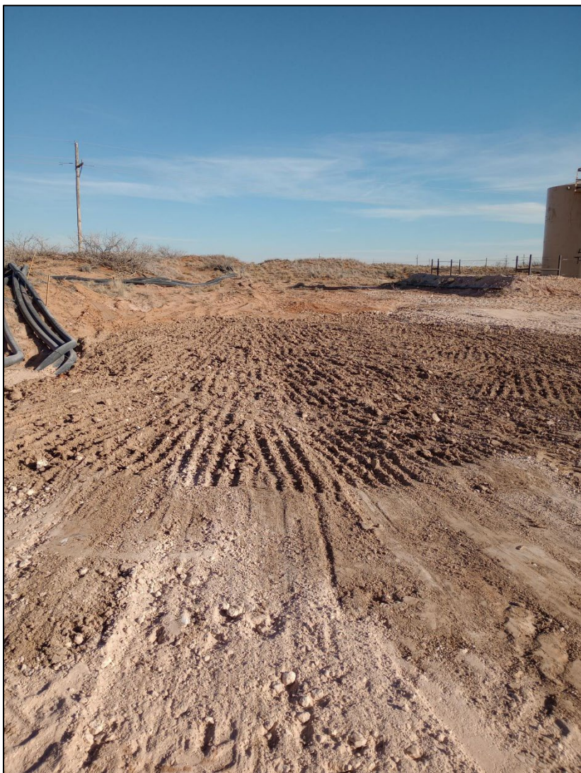
Photo 9: Area backfilled with topsoil, seeded with BLM #2 for sandy sites
