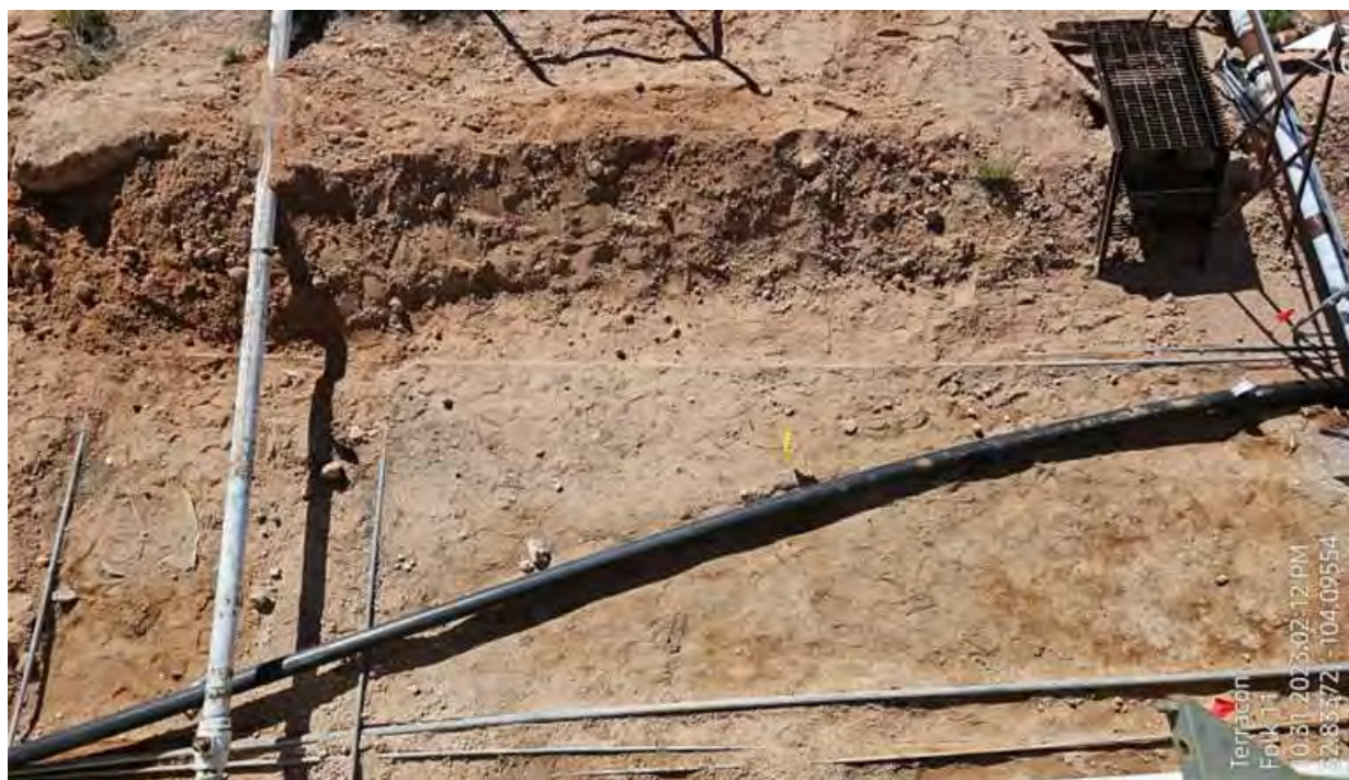
PHOTO 24: Birds eye view of the backfilled small trench on the West side of tanks.
