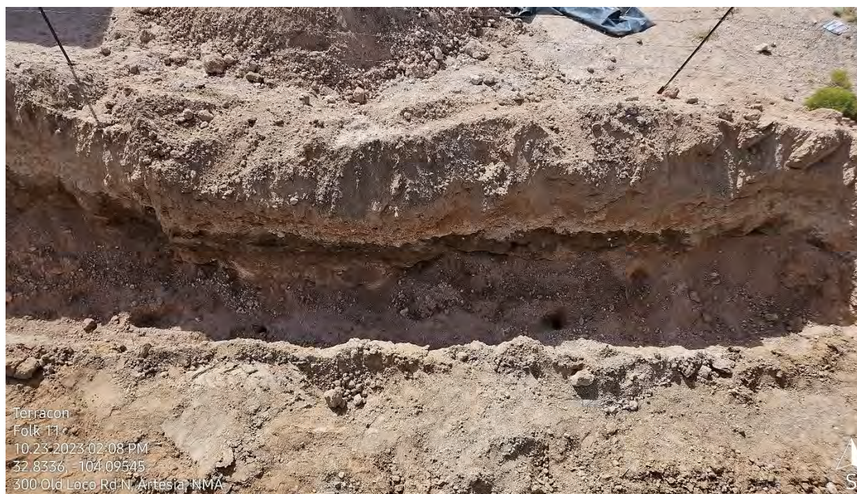
PHOTO 20: Birds eye view of the completed excavation of the West trench 2.
