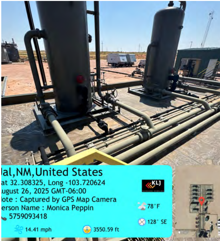
Liner under piping and vertical separators.
